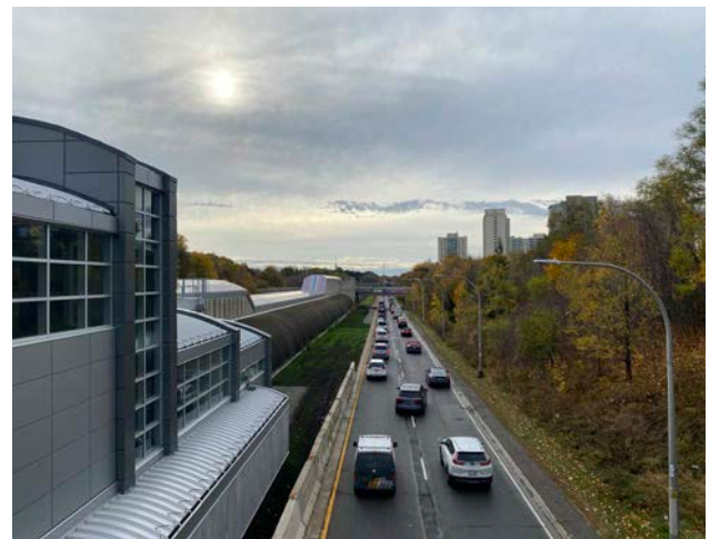
Fig. 3.12. Allen Road looking towards south, Glencairn Station to the left.
