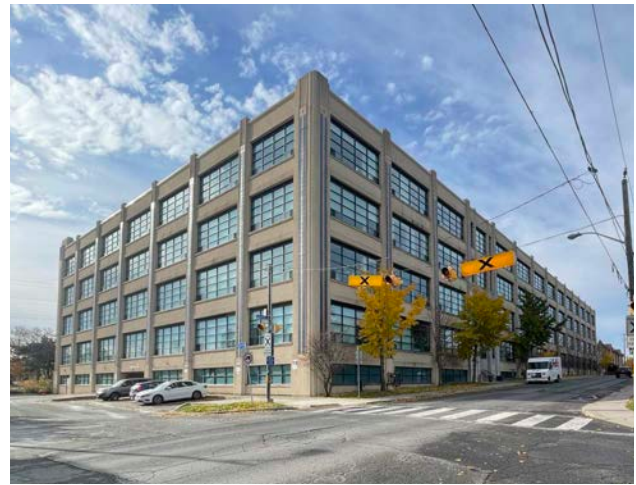
Fig. 3.7. The old Paton-Baldwin Knitting Works building (Forest Hill Lofts) located at Roselawn Avenue at Times Road, outside the study area.
