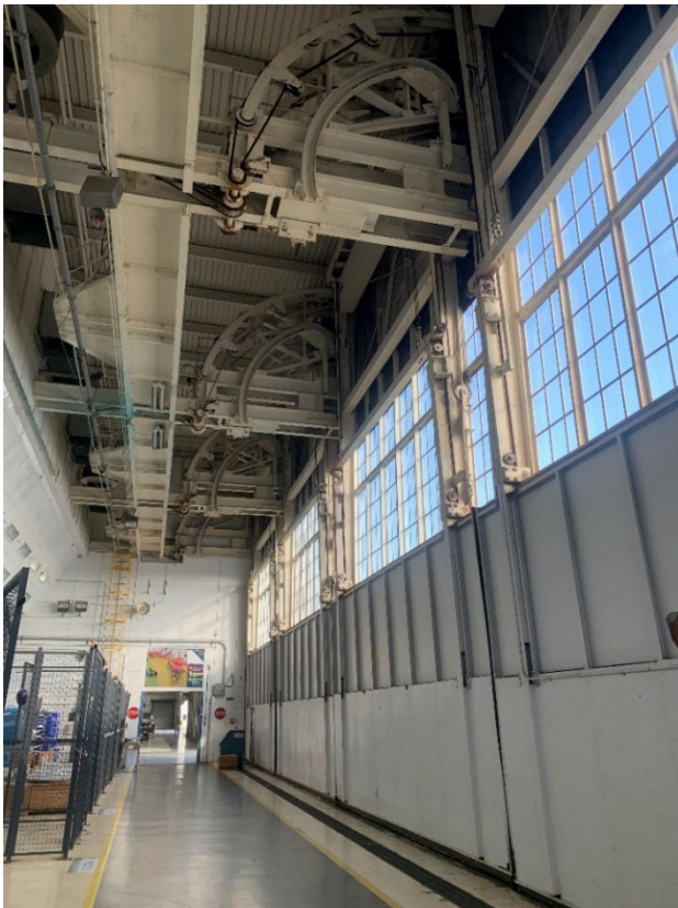
Interior view of Bay 2 and showing the overhead hangar doors with their assemblies and mechanisms. (Heritage Planning, 2023)
