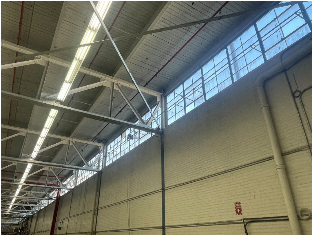
Interior of the west elevation (1953 portion) showing the pattern of ribbon windows and exposed steel ceiling trusses. (Heritage Planning, 2023)
