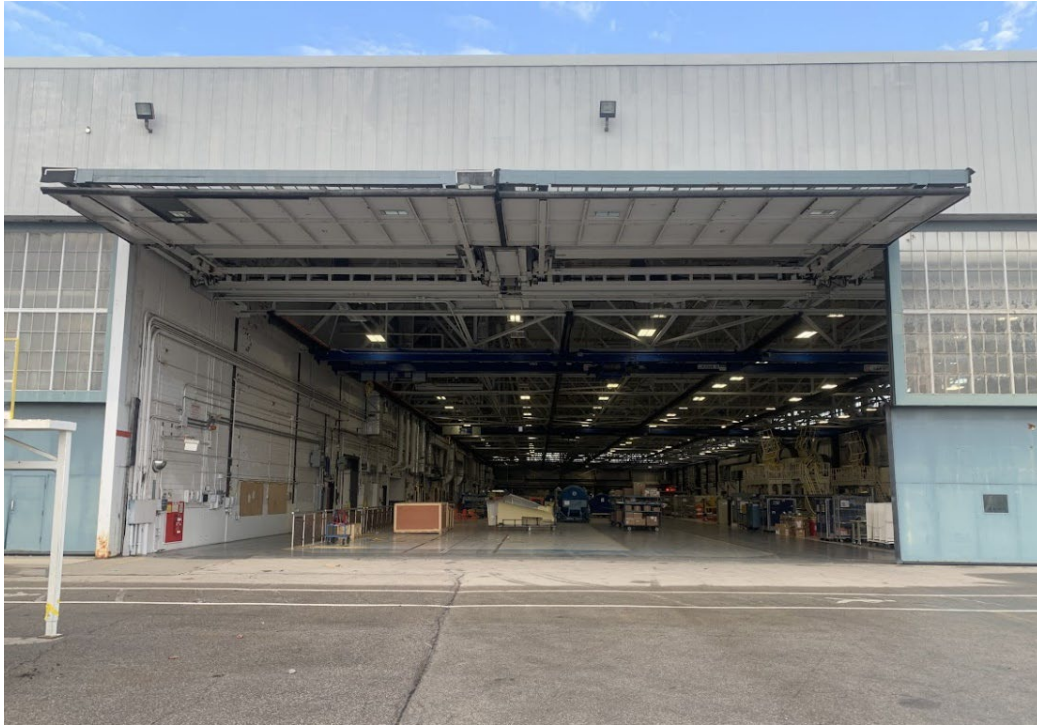
View looking west from into the interior of Bay 2 and showing the full-height interior volume with exposed steel ceiling trusses and overhead hangar door. (Heritage Planning, 2023)
