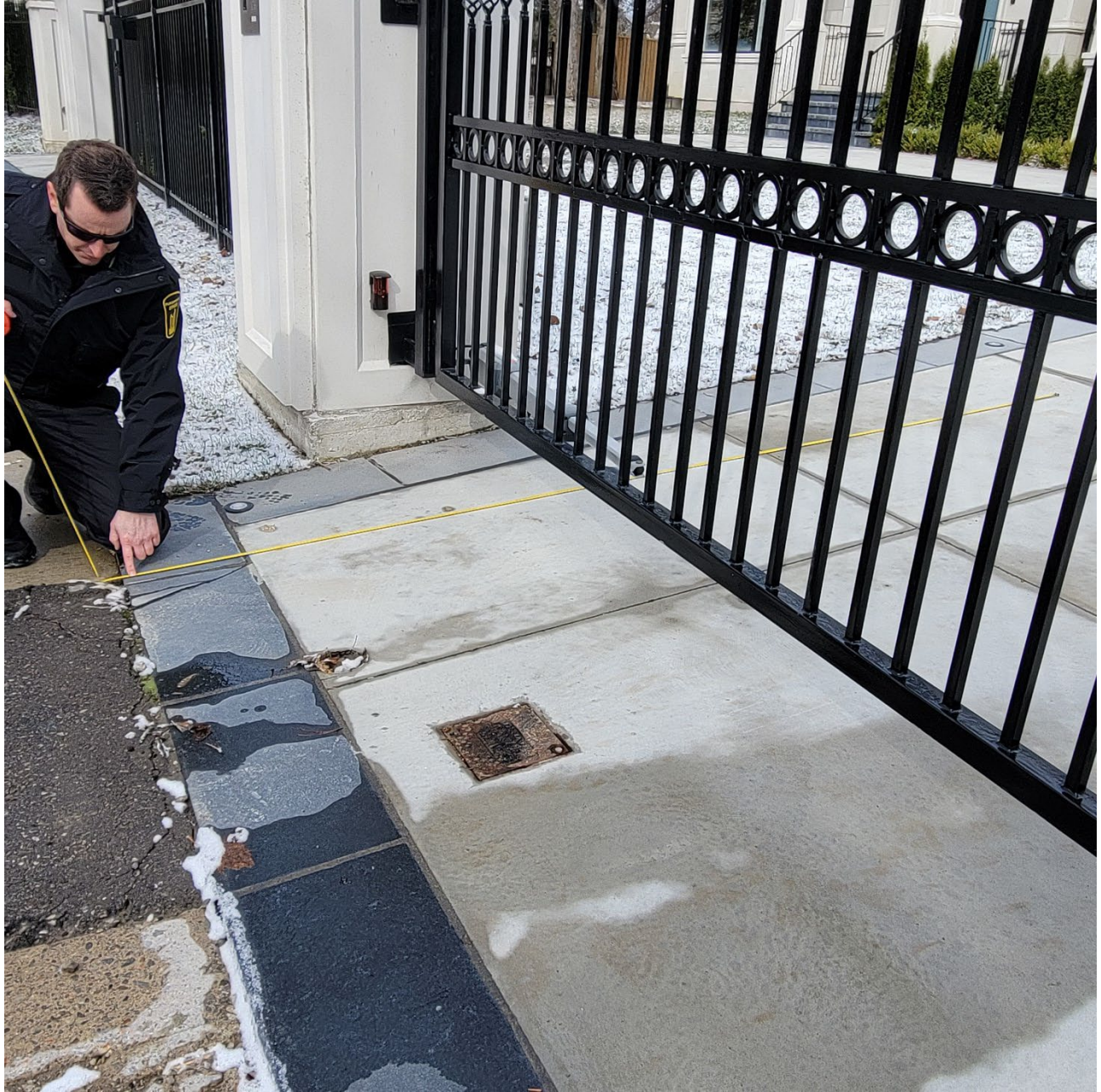
Attachment 18: Photograph depicting 2.4 metres from the front property line at the driveway at 35 Wilket Rd., this is where City of Toronto Municipal Code Chapter 447-1.2B(1) and Chapter 447-1.2C(1) applies, open-fence construction and maximum height of 1.2 metres required.
