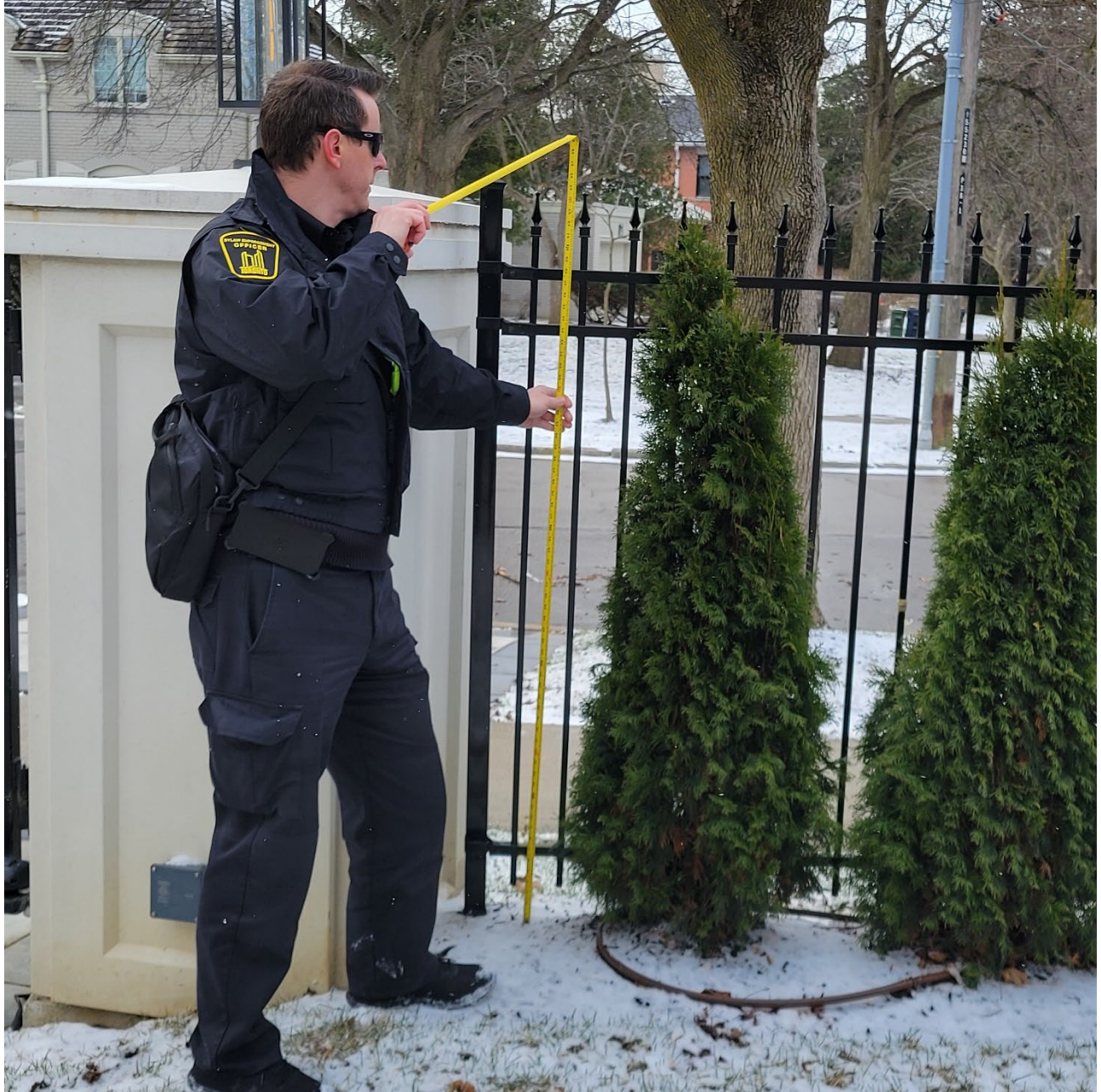
Attachment 9: Photograph depicting existing height of fence at 1.65 metres. Maximum permitted height for the fence is 1.2 metres.
