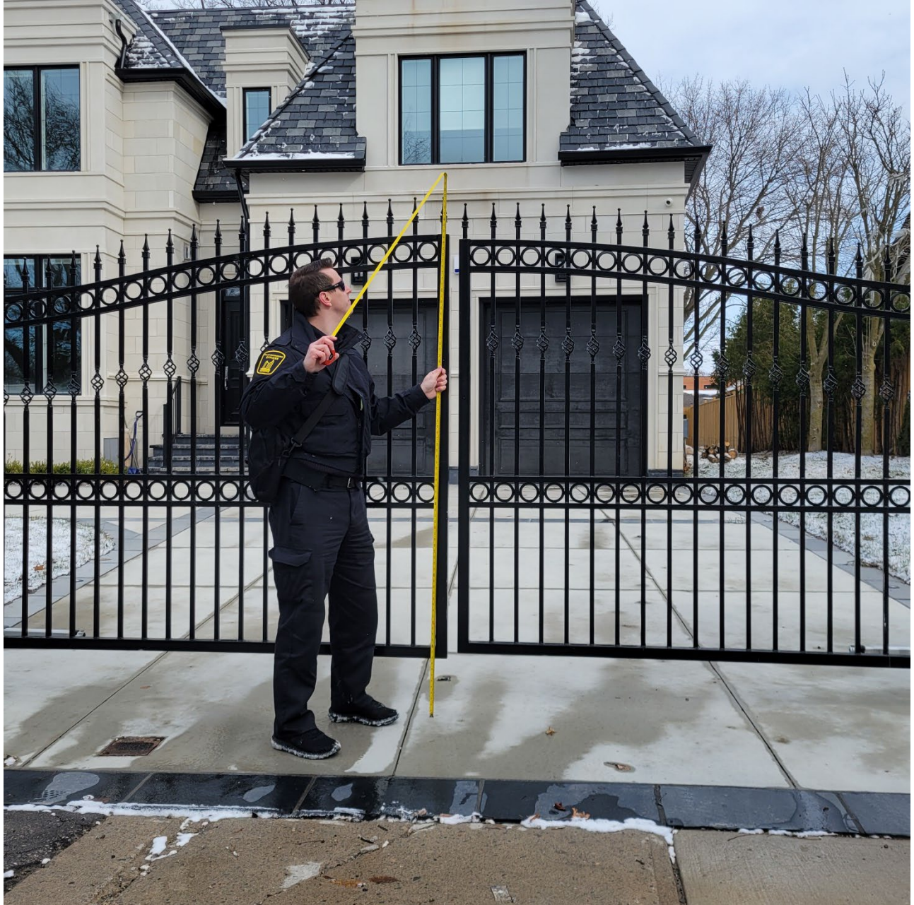
Attachment 14: Photograph depicting existing height of double swing gates at 2.22 metres. Maximum permitted height for any component of the fence is 1.2 metres.
