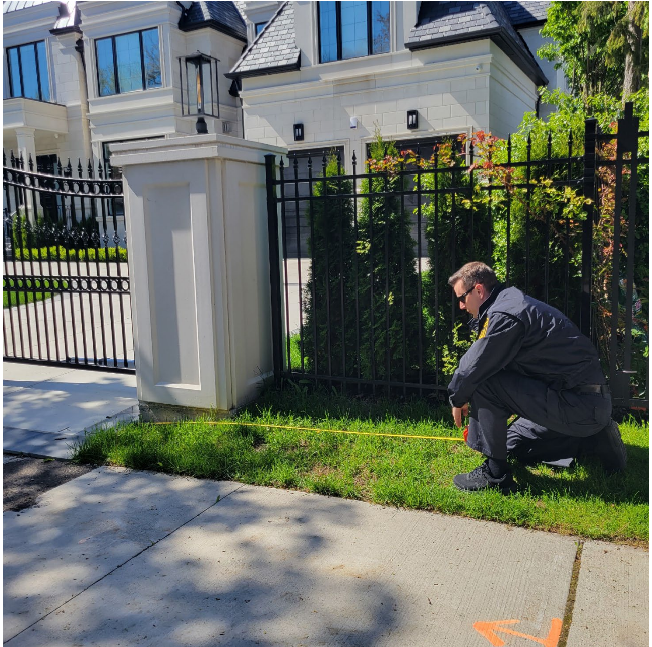
Attachment 20: Photograph depicting 2.4 metres from the driveway at 35 Wilket Rd., this is where City of Toronto Municipal Code Chapter 447-1.2C(1) applies, open-fence construction required .
