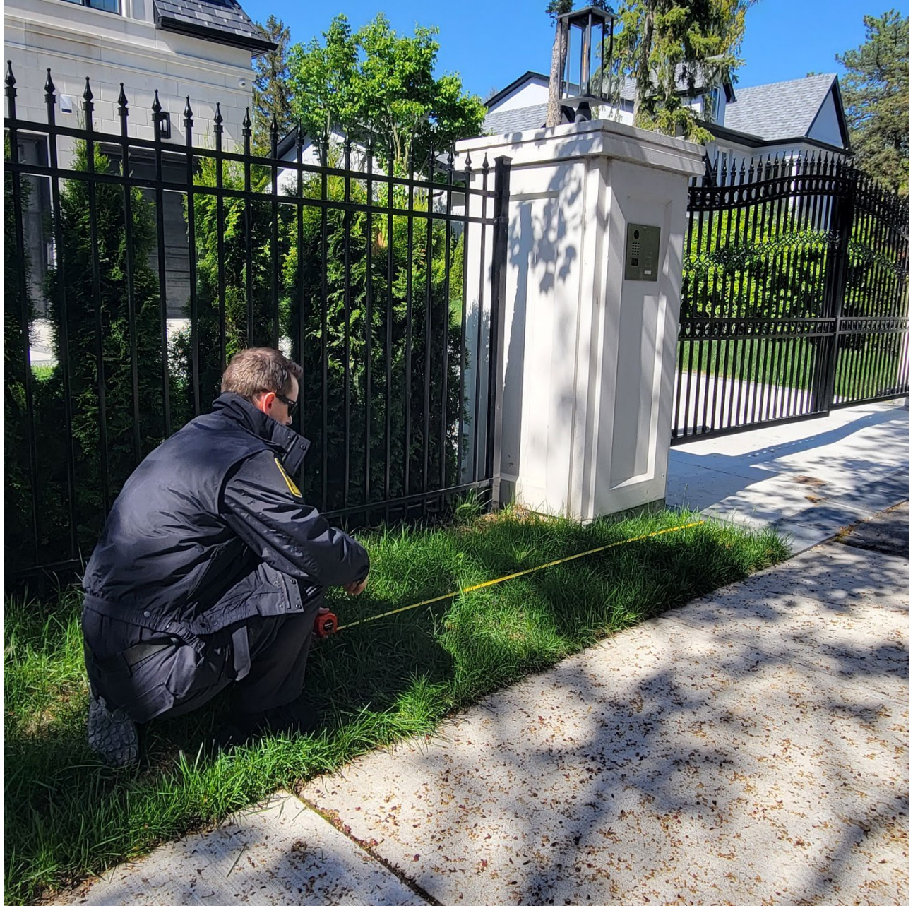
Attachment 21: Photograph depicting 2.4 metres from the driveway at 35 Wilket Rd., this is where City of Toronto Municipal Code Chapter 447-1.2C(1) applies, open-fence construction required .
