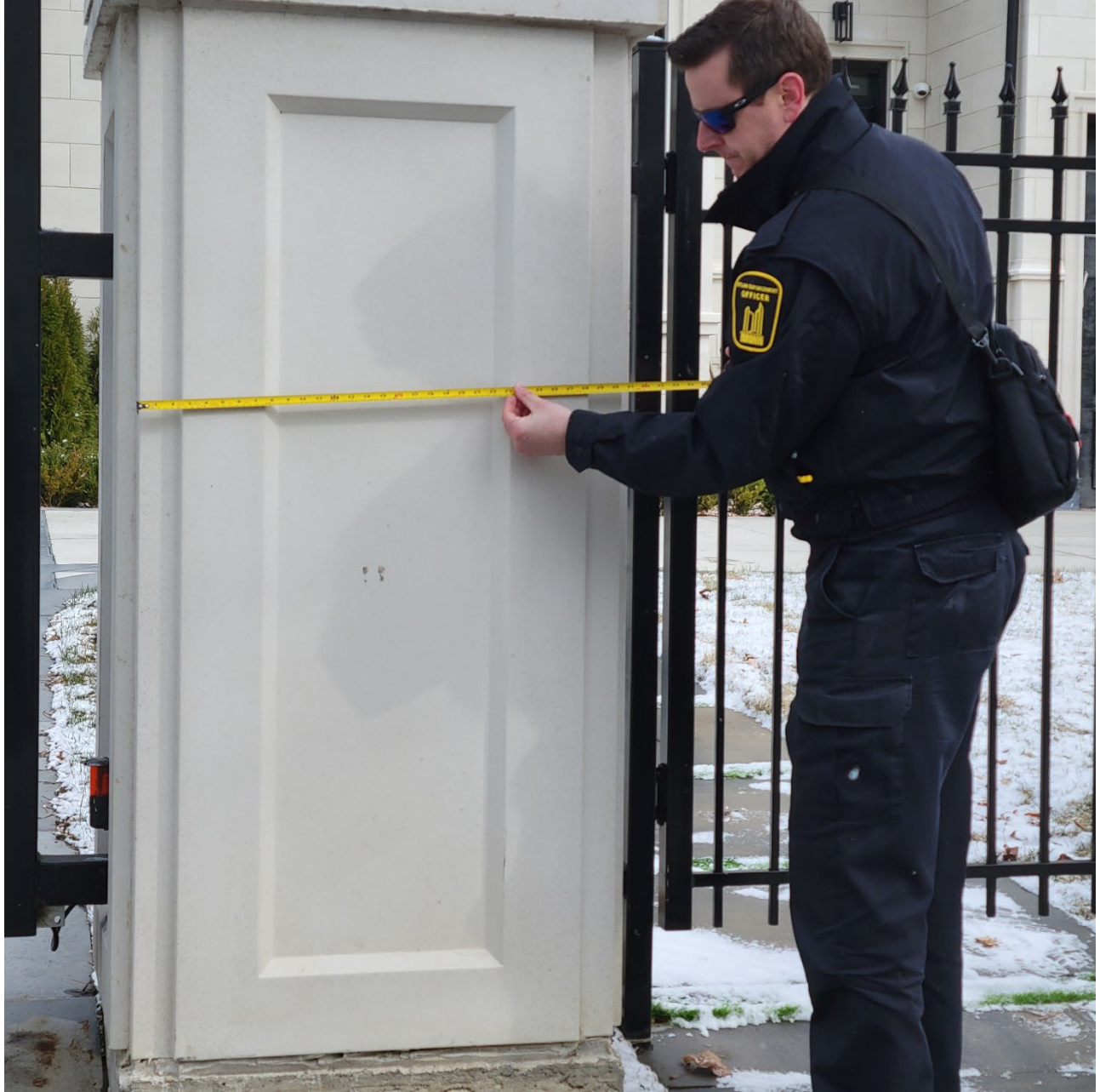
Attachment 13: Photograph depicting existing width of precast concrete columns at 0.8 metres.
