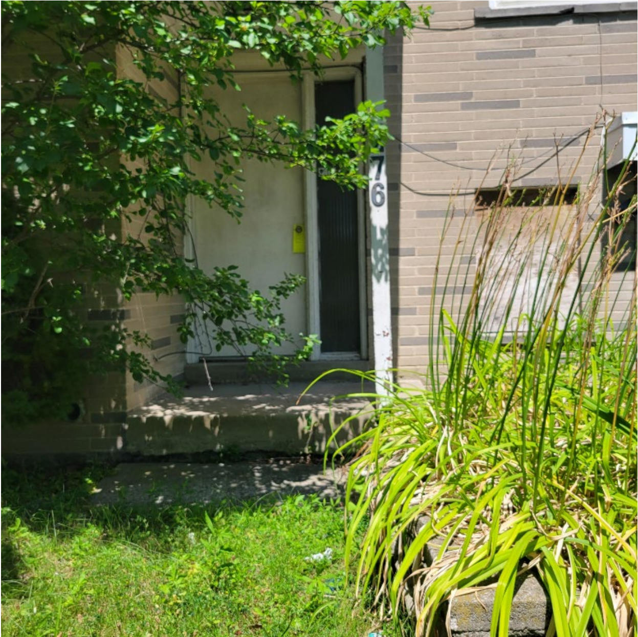
272-276 Finch Avenue East (front)
