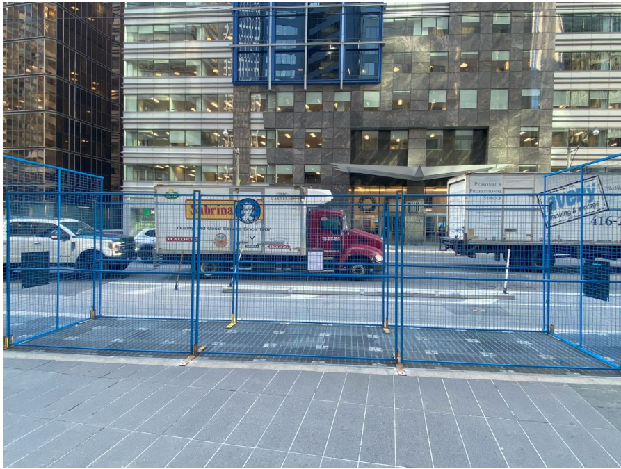
Photo 3: Fencing at University Ave. around Vent Shaft
