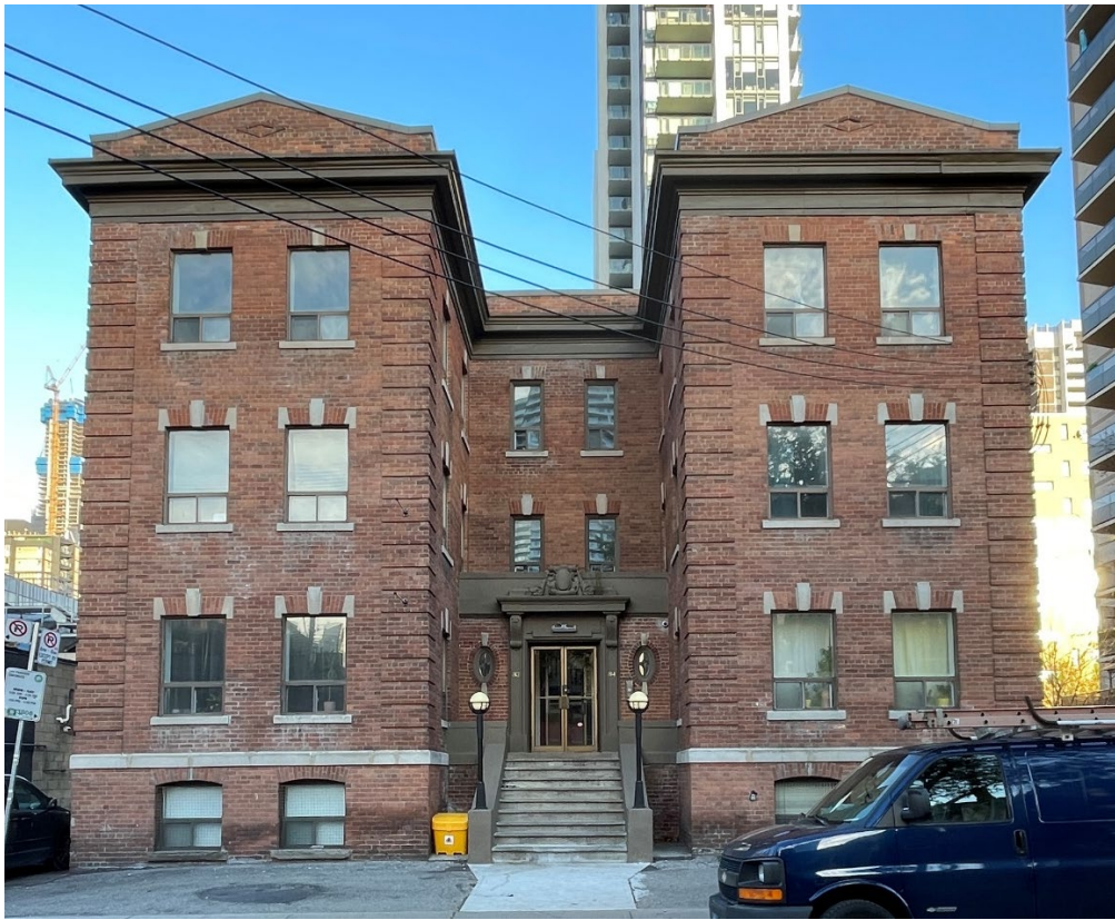
84 Maitland Street (Heritage Planning, 2024).
