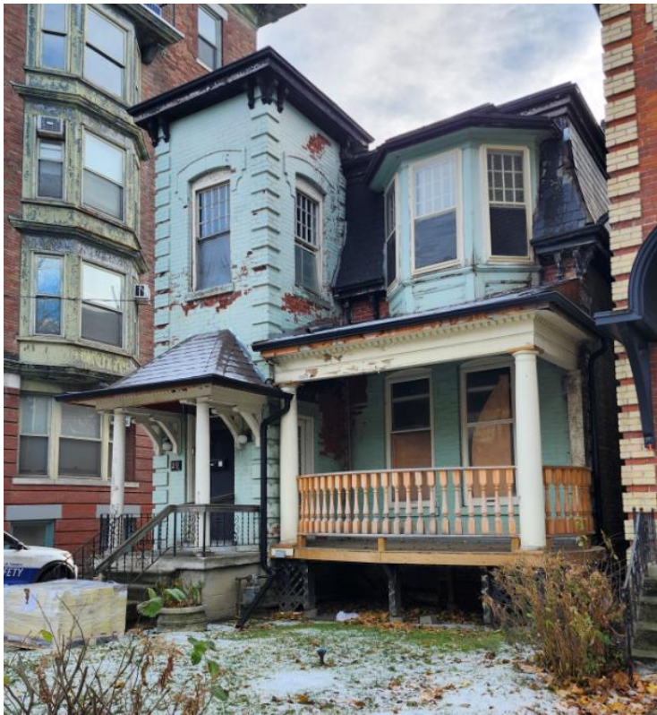
Figure 21. 29 Sussex Avenue showing the original red brick in the principal (north) elevation below the peeling paint (Heritage Planning, 2024)
