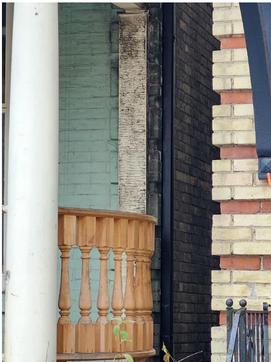
Figure 22. 29 Sussex Avenue showing the original buff brick chaine at the northwest corner that is not concealed by paint (Heritage Planning, 2024)
