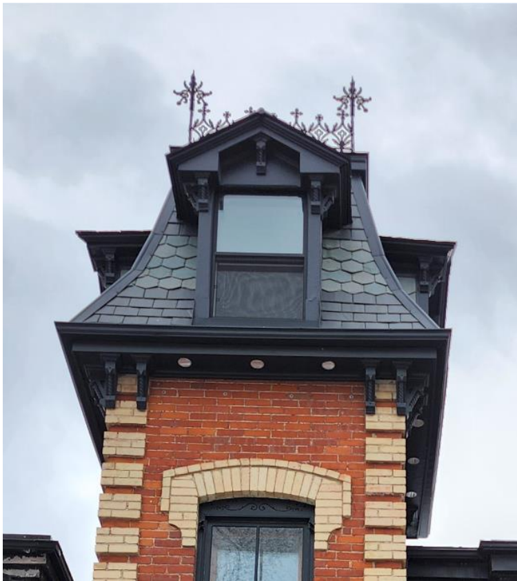
Figure 12. 31 Sussex Avenue showing the mansard roof of the tower with its patterned slates, dormer windows with pediments and iron cresting (Heritage Planning, 2024)
