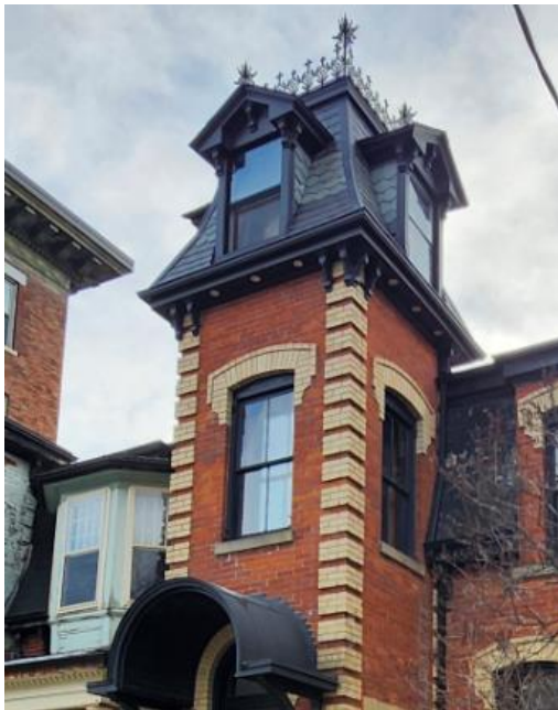
Figure 16. 31 Sussex Avenue showing the details on the tower including the chaine at the corners, the pierced wood lintel over the windows and the paired brackets at the eaves (Heritage Planning, 2024)
