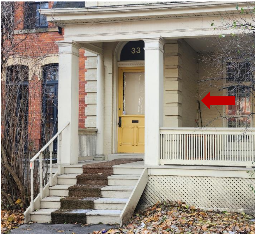
Figure 20. 33 Sussex Avenue showing the chaine extending to the tower return (Heritage Planning, 2024)
