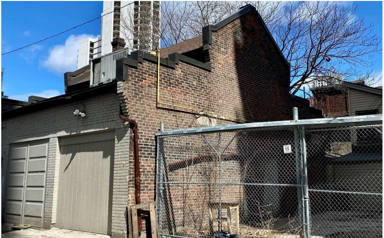
The rear coach house, viewed from Donna Shaw Lane, 2022 (Heritage Planning).
