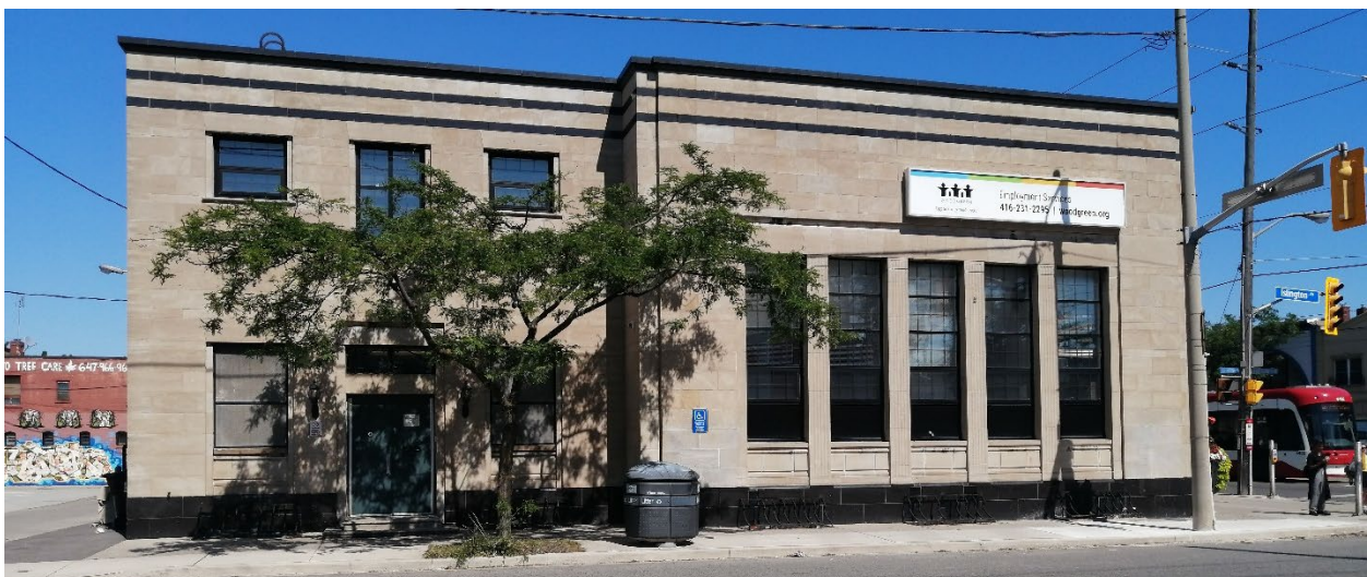
Figure 4 Looking east from Islington Avenue towards the west elevation of 1935 structure's main and rear wings (Heritage Planning, 2024).
