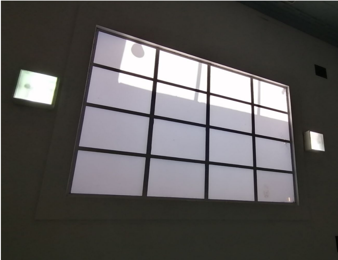
Figure 14 Interior image of the postal hall skylight (Heritage Planning, 2024).
