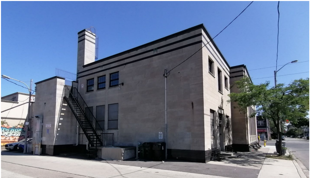
Figure 7 Looking southeast from the rear laneway off Islington Avenue towards the rear and west elevations of the 1935 structure (Heritage Planning, 2024).
