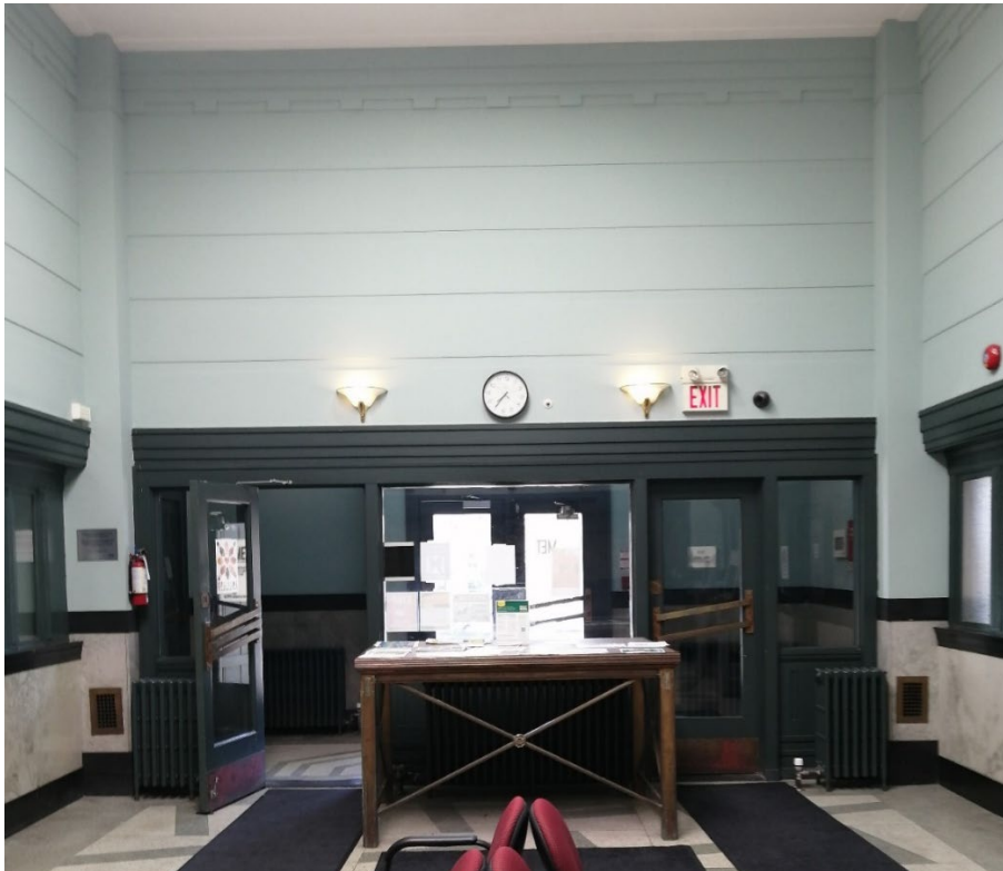
Figure 10 Interior image of the postal hall looking south towards the vestibule showing original doors, plasterwork, terrazzo floors, marble dado, and brass postal table (Heritage Planning, 2024).
