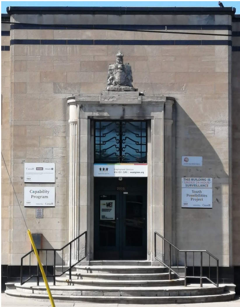
Figure 3 Detail of central entrance with double entrance, transom with iron grille, semi circular stairs, and door surround featuring columns and Coat of Arms of Canada (Heritage Planning, 2024).
