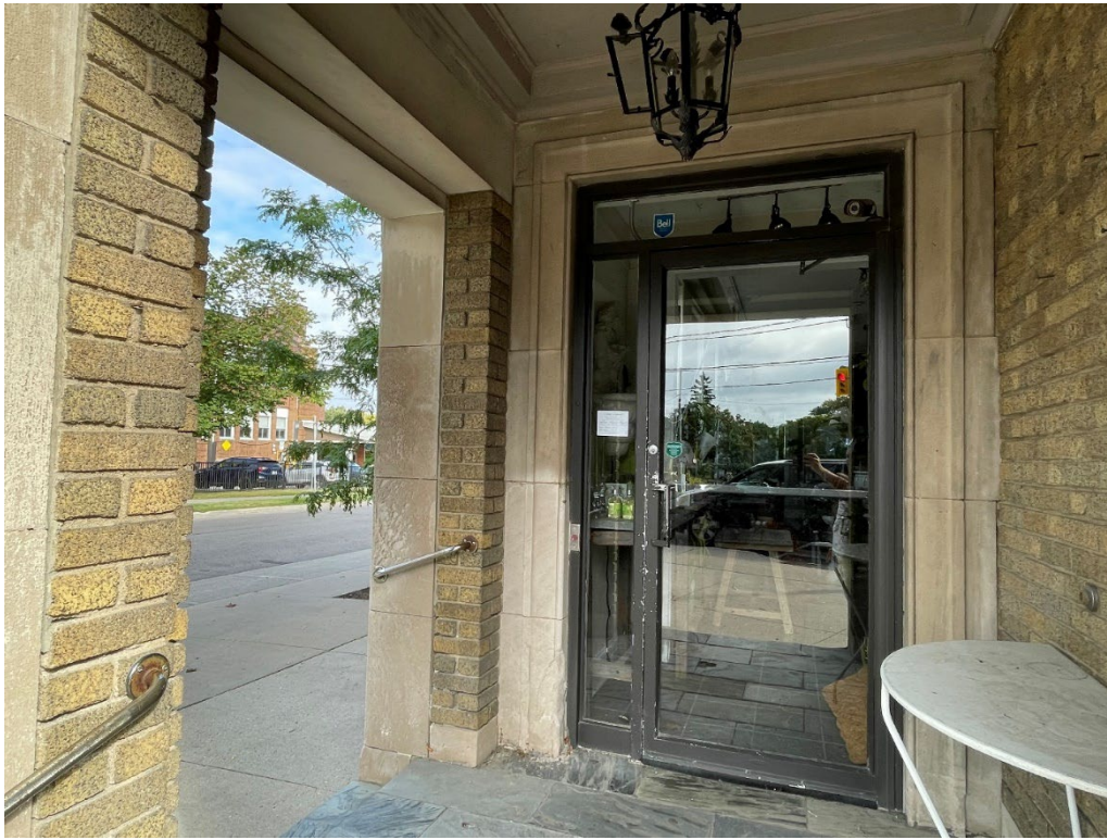
Figure 9: integral main entrance, 2024 (City of Toronto Heritage Planning)
