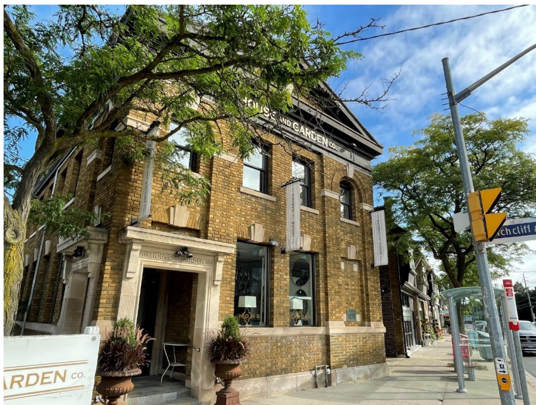
View from the west of 1660 Kingston Road, 2024 (City of Toronto Heritage Planning)
