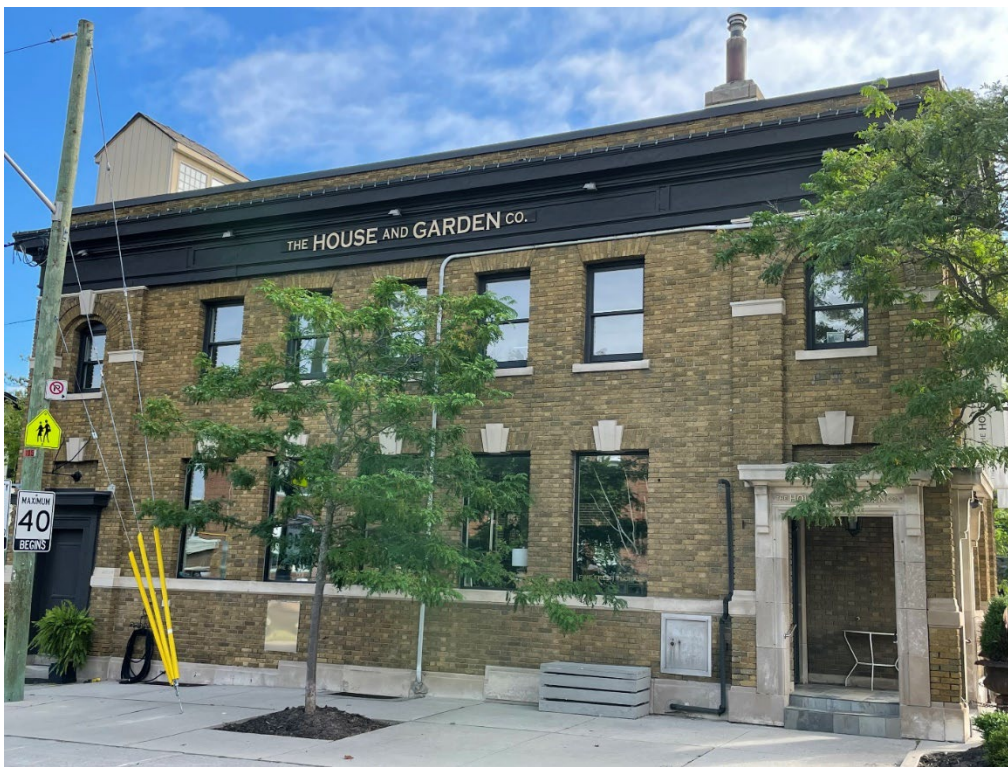
Figure 6: view from the southwest showing the west façade, 2024 (City of Toronto Heritage Planning)
