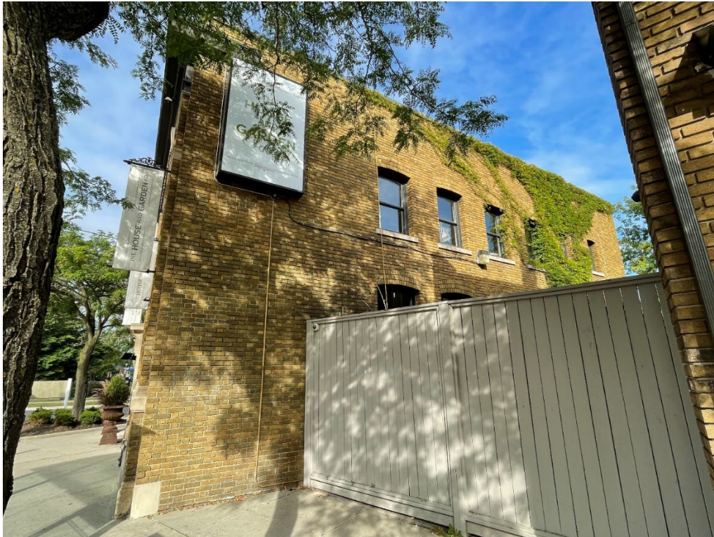
Figure 10: view from the southeast showing the east façade, 2024 (City of Toronto Heritage Planning)
