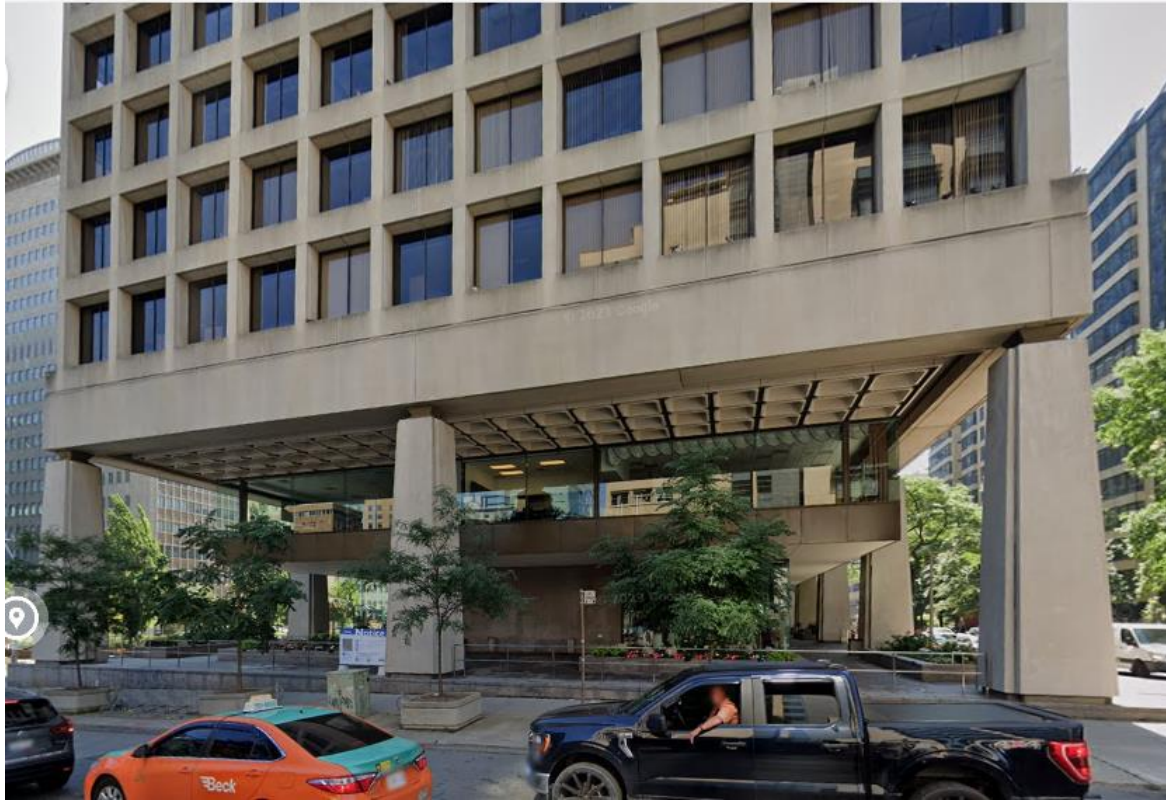
Close up view of ground floor plane
