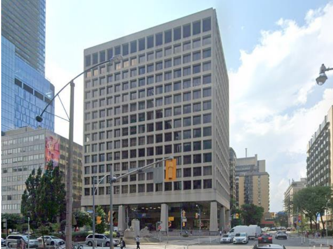
View of property from intersection of University Ave and Elm St
