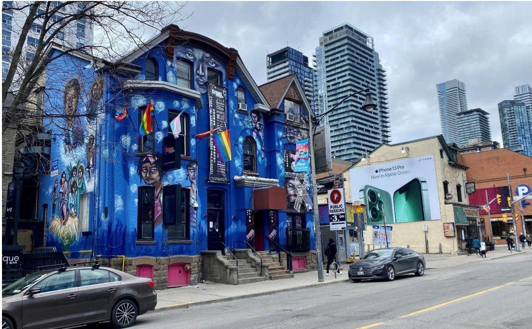
Northwestward view of the subject properties from across Church Street, 2022 (Heritage Planning).
