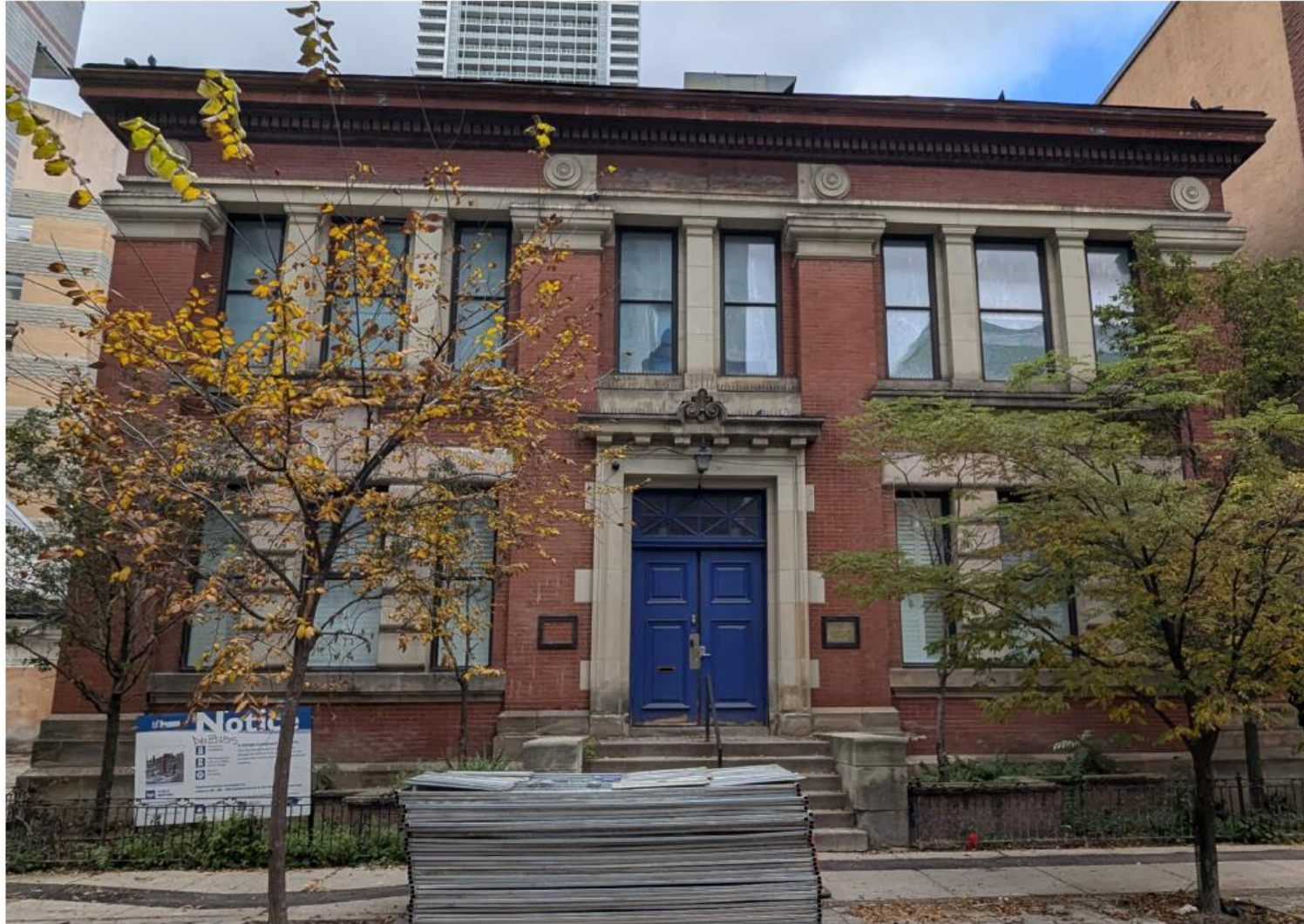
South (principal) elevation of 86 Lombard Street (ERA Architects Inc., 2024).
