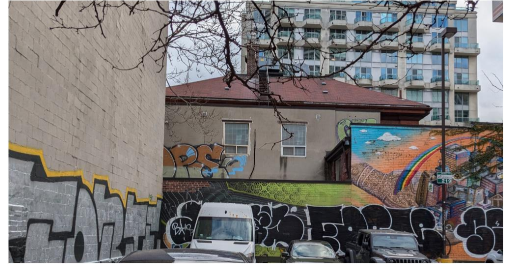
North (rear) elevation (ERA Architects Inc., 2024).
