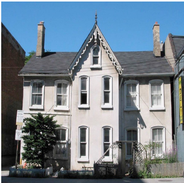
122-124 Peter Street (buildings now demolished following a fire in 2018).
