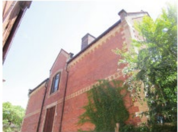
North elevation of 349 George Street (ERA)
