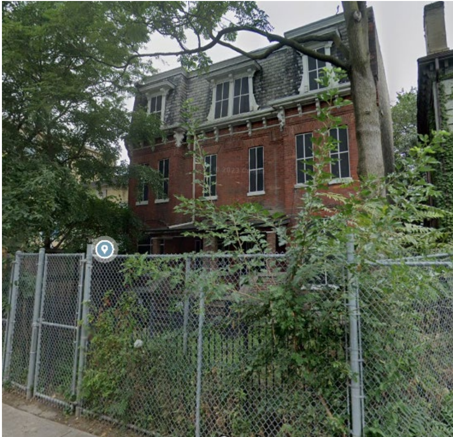
309-311 George St - west elevation (Google Maps 2023)
