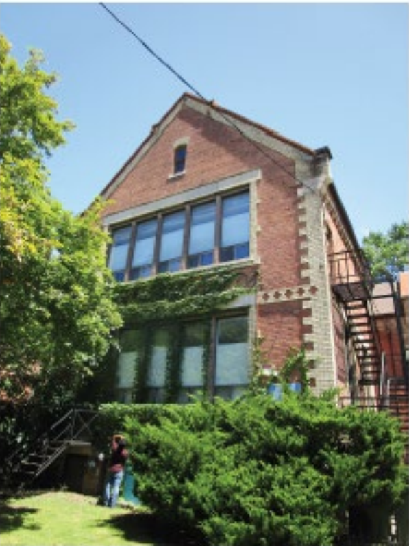
West elevation of 349 George Street (ERA)
