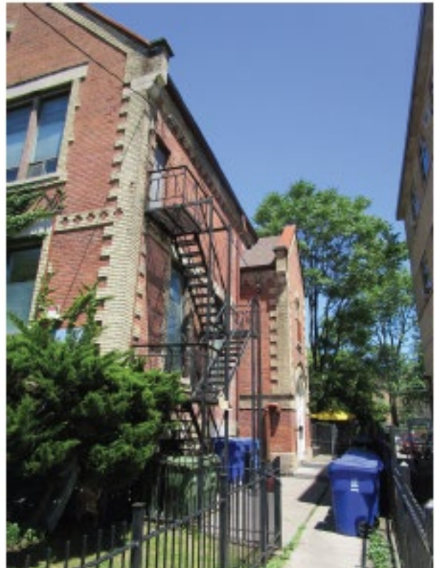
South elevation of 349 George Street (ERA)
