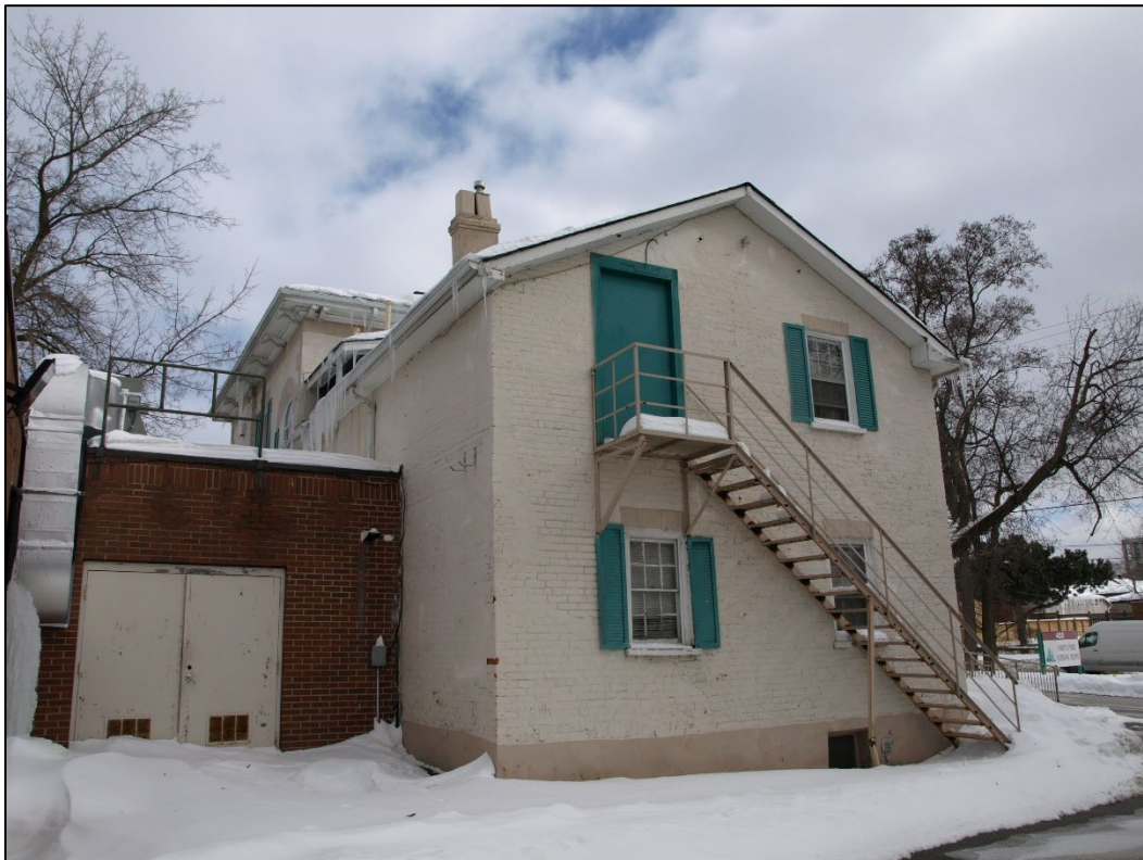
Figure 23: Downs View House, west elevation. (Heritage Planning, 2025)
