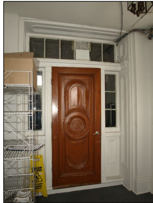
Figures 28 and 29: Left: On the first floor of the c. 1855 section's two-storey projecting tower, lie one of the two painted windows. Right: Same area, the historic structure's intact formal front entryway, including its ornately carved wooden door, transom, sidelights, and surround. (Fayle Associates, 1994, and Heritage Planning, 2025 respectively)
