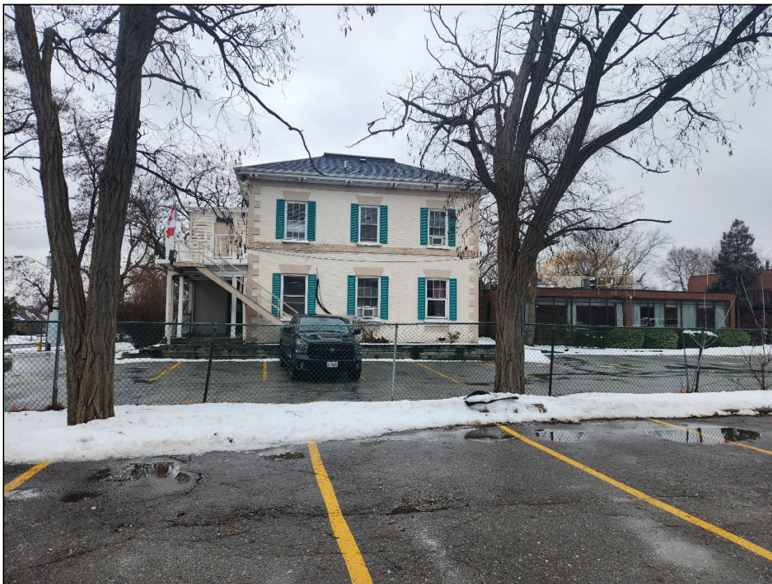
Figure 21: Downs View House, east elevation. (Heritage Planning, 2025)
