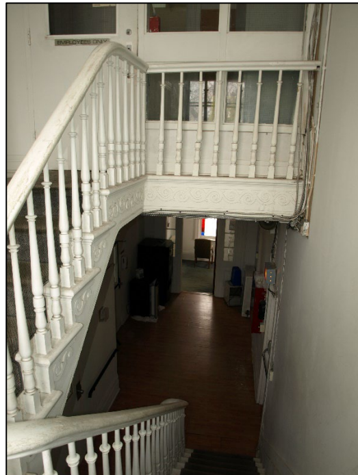
Figures 30 and 31: Left: the c. 1855 section's J-Plan, or double-winder, stairway, and its side-hall plan layout. Right: On the landing looking south towards the first and second floors of the two-storey projecting tower (c. 1855 section). Visible in the distance is one of the two painted-glass windows, located on the first floor of the tower. (Heritage Planning, 2025)
