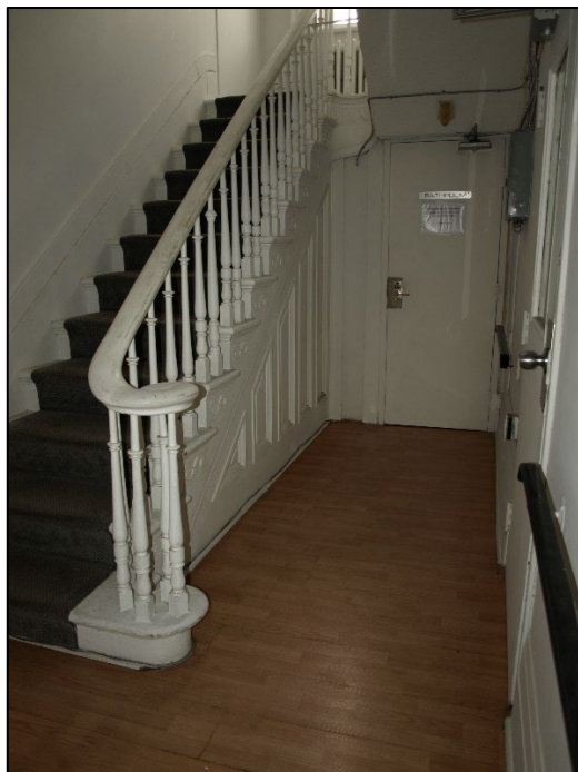
Figures 30 and 31: Left: the c. 1855 section's J-Plan, or double-winder, stairway, and its side-hall plan layout. Right: On the landing looking south towards the first and second floors of the two-storey projecting tower (c. 1855 section). Visible in the distance is one of the two painted-glass windows, located on the first floor of the tower. (Heritage Planning, 2025)
