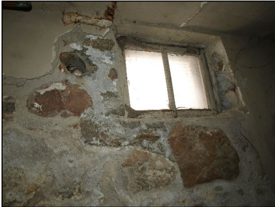
Figures 35 and 36: Left: Detail of the c. 1843 fieldstone foundation wall, taken from inside the building. Right: Detail of the c. 1855 fieldstone foundation wall, under the verandah floor. (Heritage Planning, 2025)
