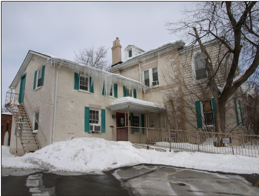
Figure 22: The c. 1843, Georgian influenced section of Downs View House likely started out as a balanced three-bay configuration, with a fourth, six-over-three window on the east side of the second floor. (Heritage Planning, 2025)
