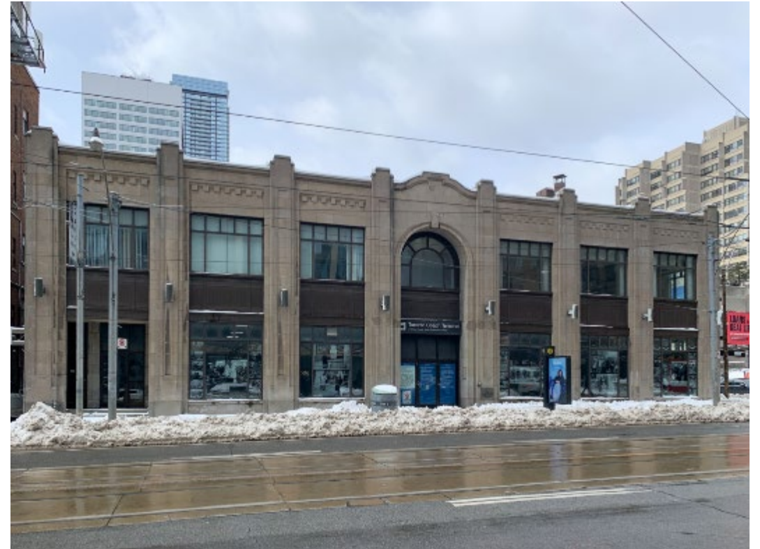
604 Bay Street – east elevation (Heritage Planning, 2025)
