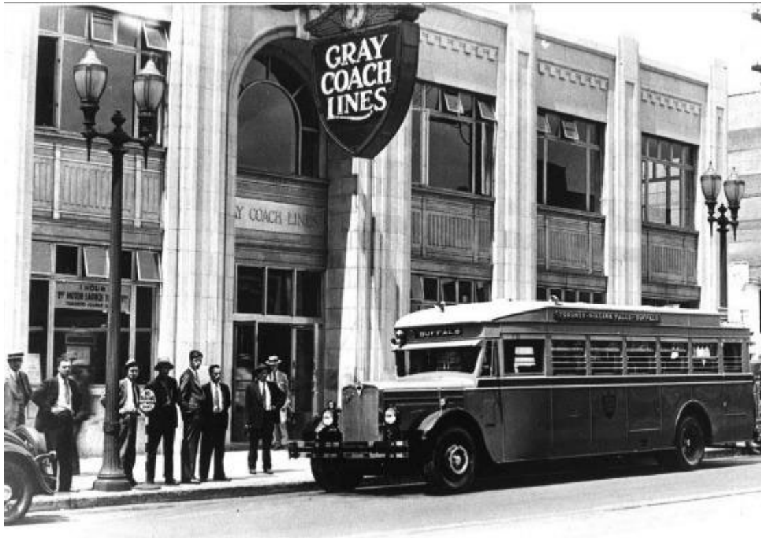
604 Bay Street – east elevation, 1932 (City of Toronto Archives)
