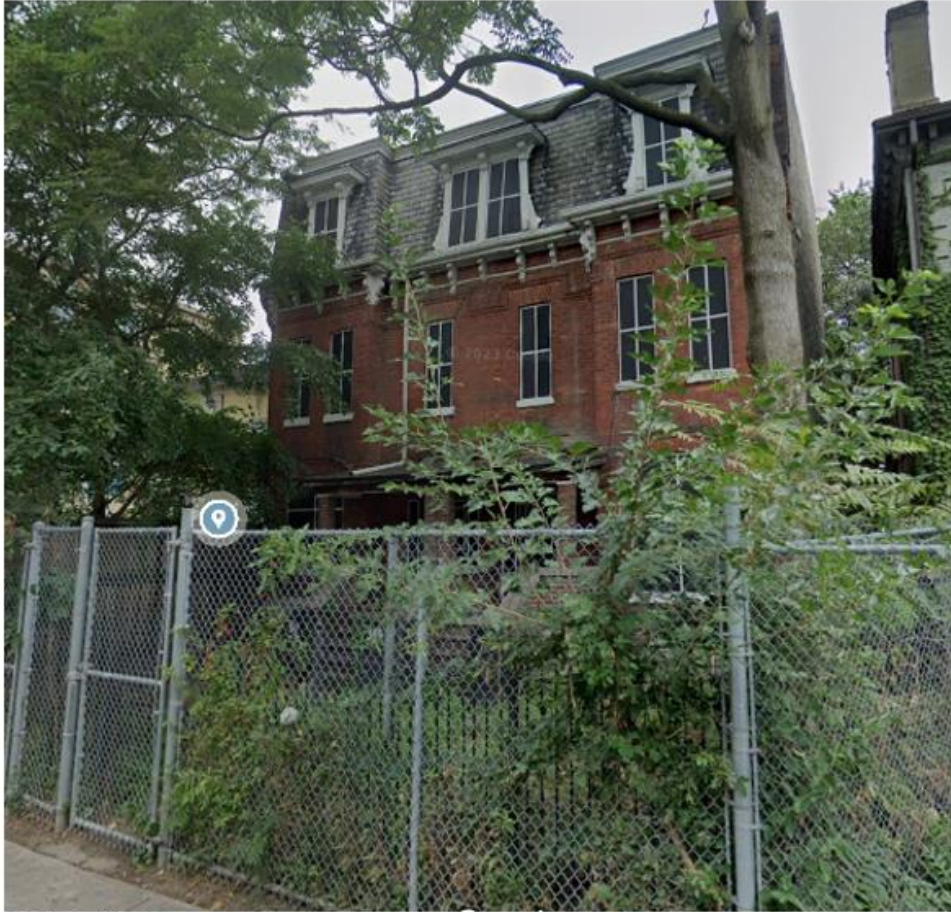
309-311 George St - west elevation (Google Maps 2023)
