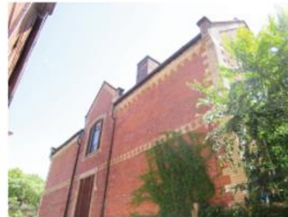
North elevation of 349 George Street (ERA)
