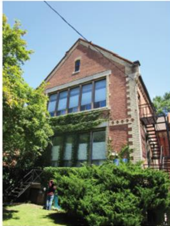
West elevation of 349 George Street (ERA)
