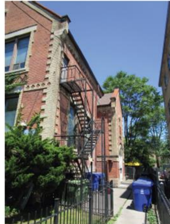
South elevation of 349 George Street (ERA)
