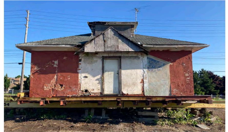
The south (rear) elevation of 5951 Steeles Avenue East looking north (ERA Architects Inc., 2024).
