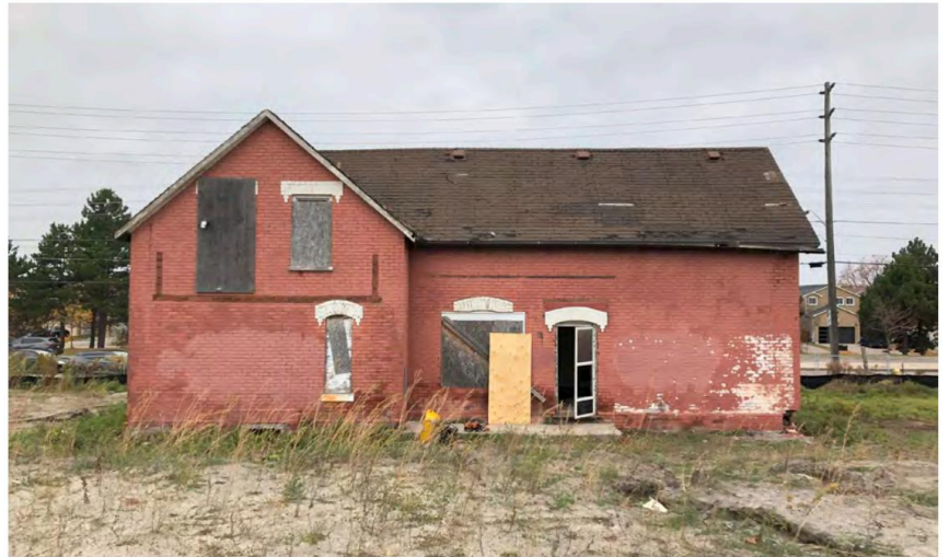
The south (rear) elevation of 5933 Steeles Avenue East looking north (ERA Architects Inc., 2024).
