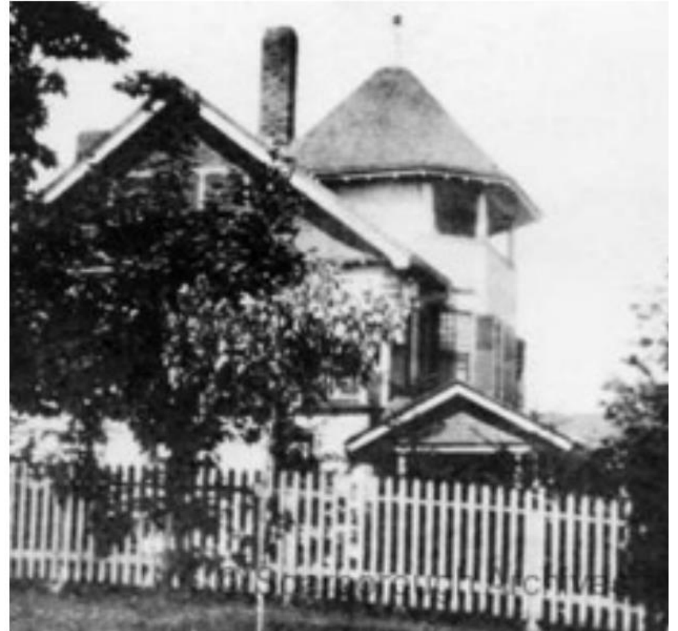
View of the west and south elevations looking east, showing the former turret at the south elevation (date unknown) (Scarborough Archives).
