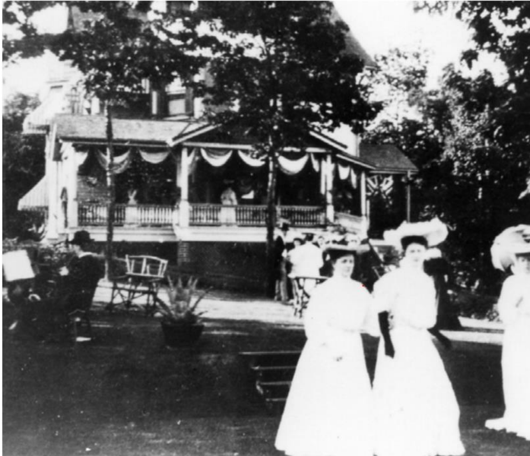
Archival photograph of the south elevation, showing the original porch condition (date unknown) (Scarborough Archives).
