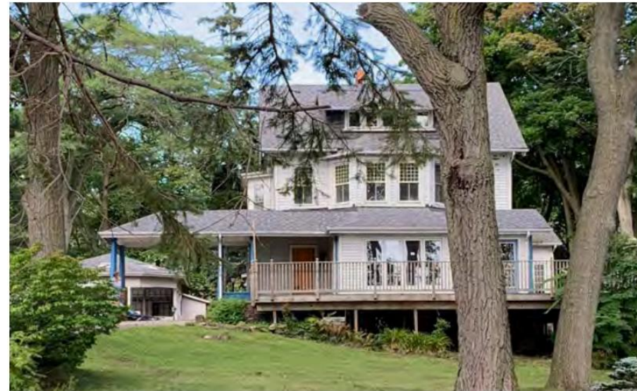
South elevation of 1 Fallingbrook Road, looking north (ERA Architects Inc.).
