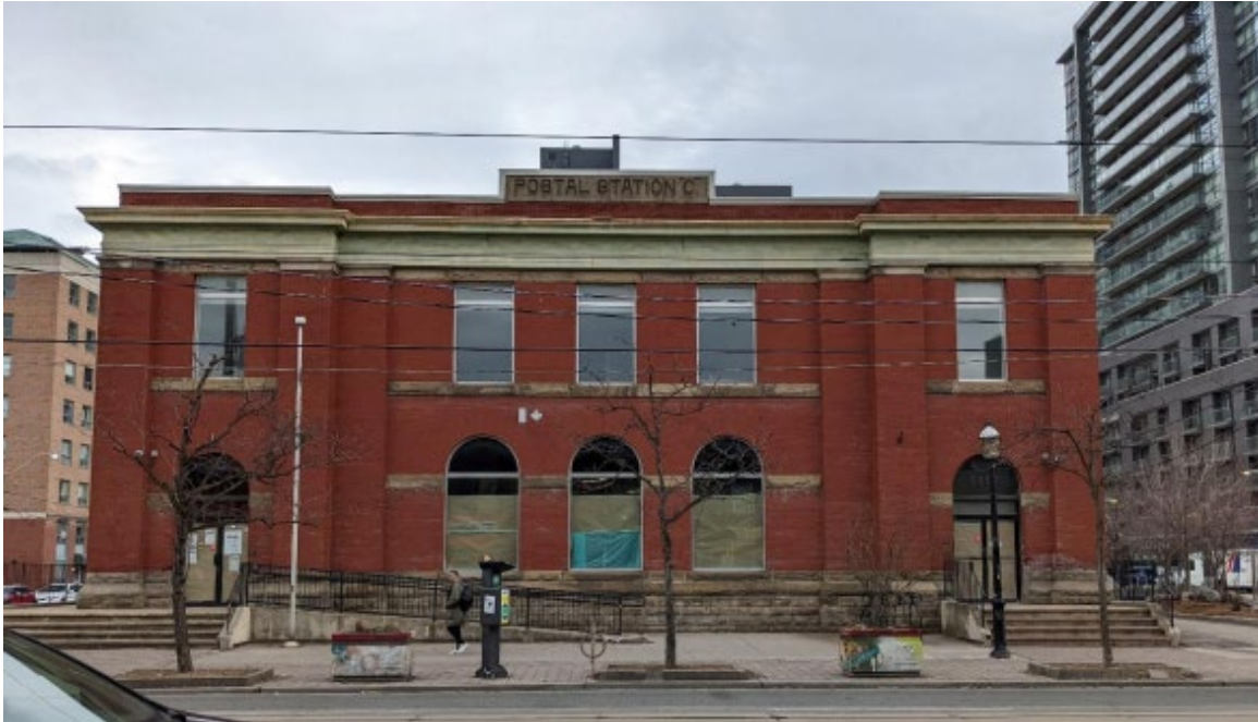
Principal (north) Elevation fronting Queen St W
