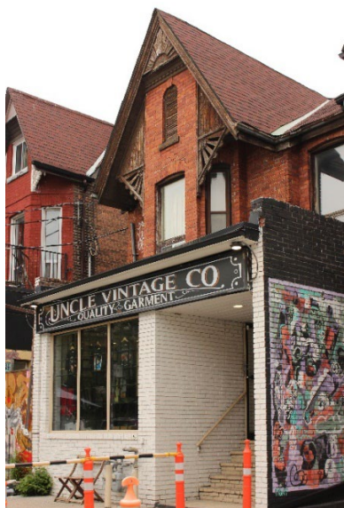
Figure 19. 33 Kensington Avenue one-storey storefront detail (Heritage Planning, 2025)
