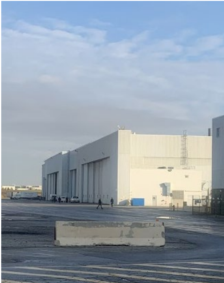
West elevation of Bays 7-10. (Heritage Planning, 2023)
