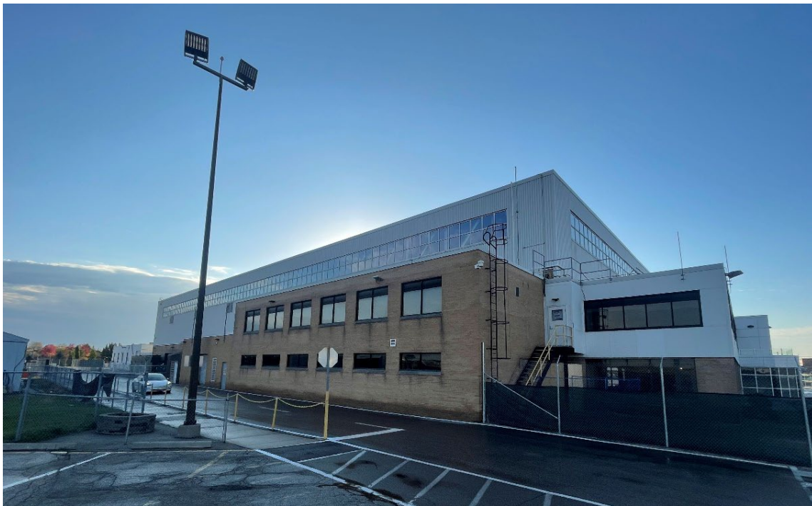
North elevation of Bay 12. (Heritage Planning, 2023)
