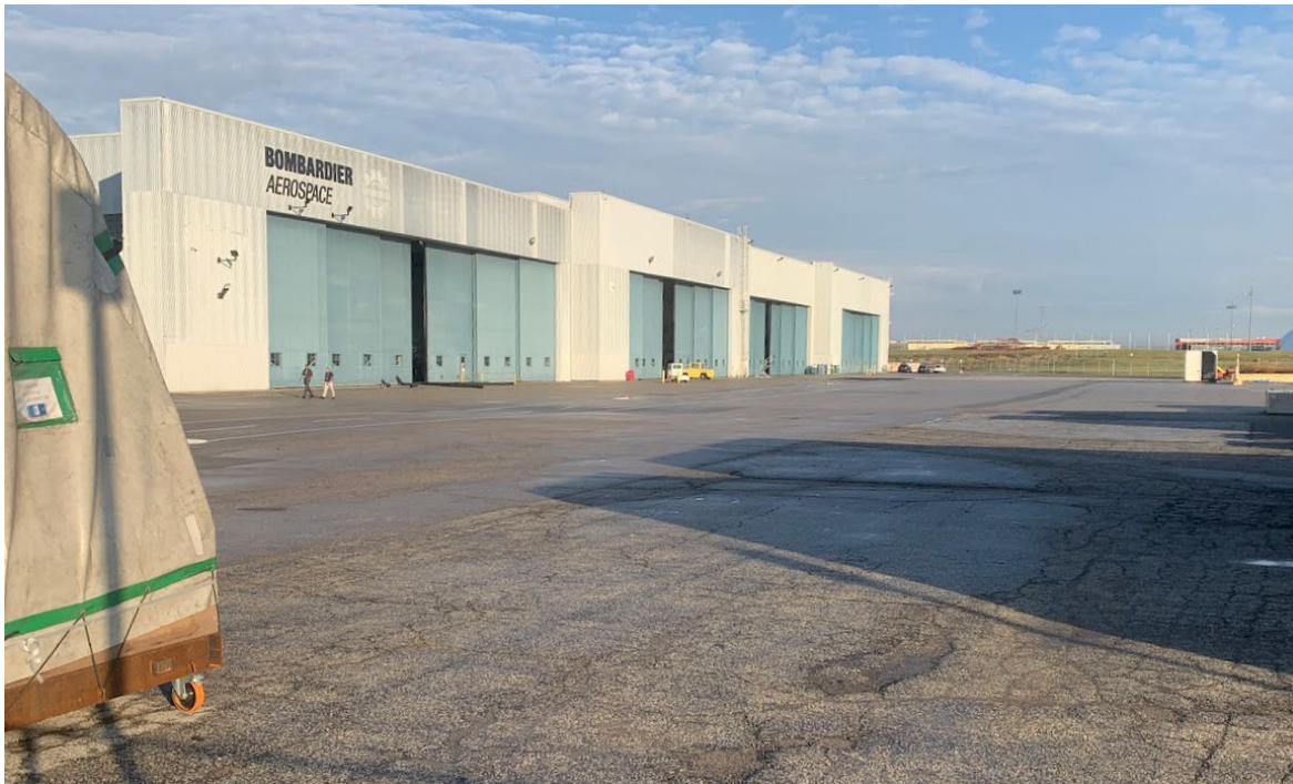
East elevation of Bays 7-10. (Heritage Planning, 2023)
