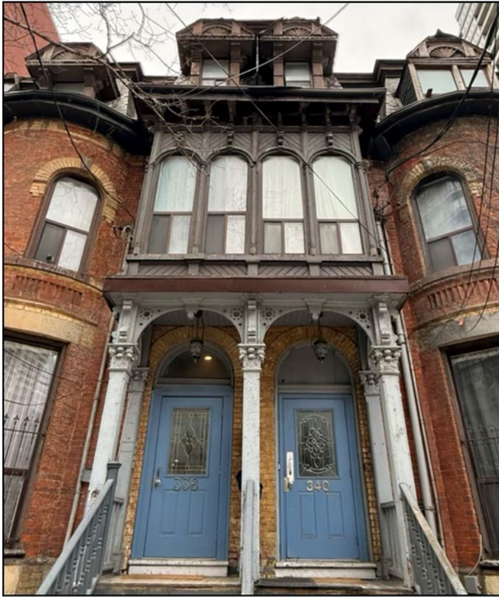
Figure 19. Detail of the primary entrances to 338 and 340 Jarvis Street, showing the second storey sunroom and columns (Alex Corey Heritage Consulting, 2025).
