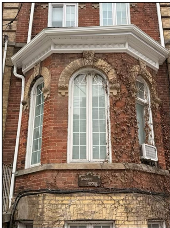
Figure 23. First storey bay window on 344 Jarvis Street (Alex Corey Heritage Consulting, 2025).
