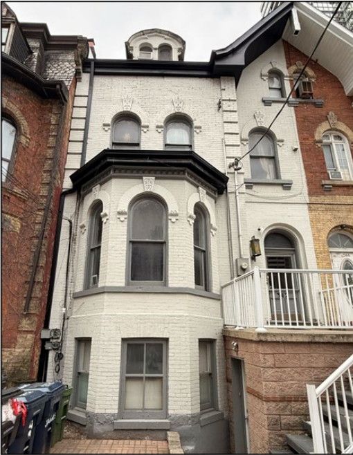
Figure 25. Primary (west) face of 342 Jarvis Street showing ornamentation that has been painted over (Alex Corey Heritage Consulting, 2025).
