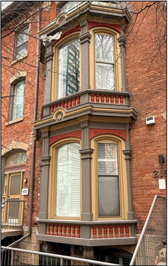
Figure 25. Two-storey bay window detail at 213 Jarvis Street (Alex Corey Heritage Consulting, 2025).
