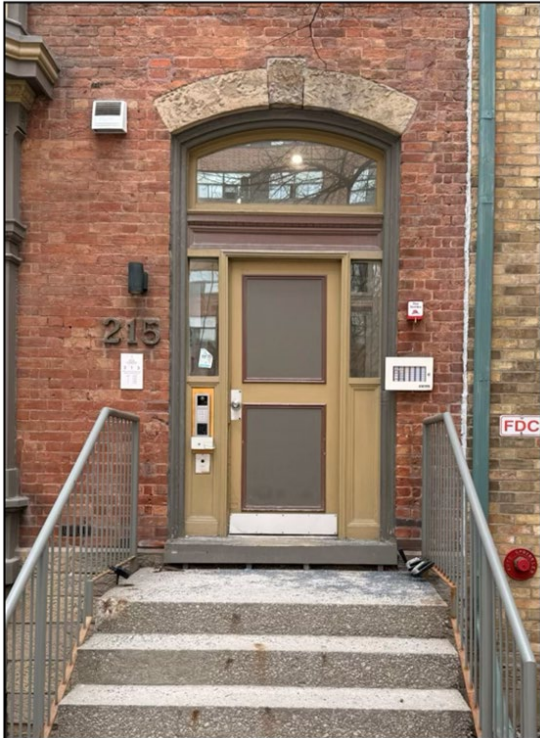
Figure 24. Entrance detail to 215 Jarvis Street (Alex Corey Heritage Consulting, 2025).
