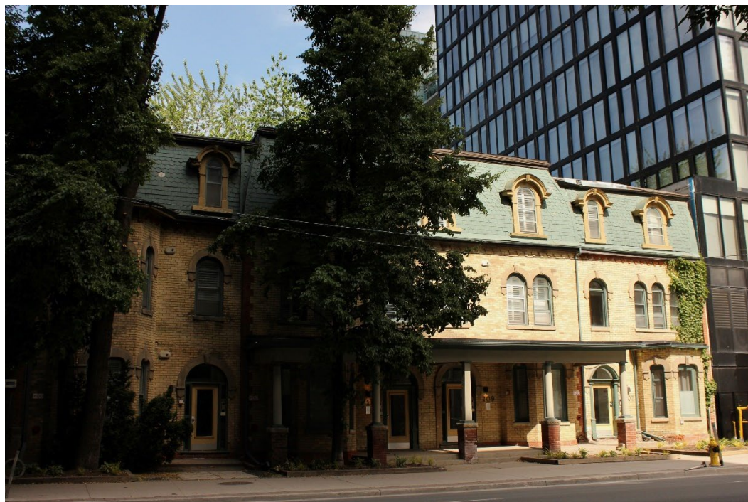
Figure 2. From right to left: 207, 209, 211, and 213 Jarvis Street (Heritage Planning, 2025).
