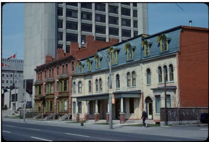
Figure 17. Jarvis Street, north of Shuter Street, subject properties, east side, 1979 (CTA).
