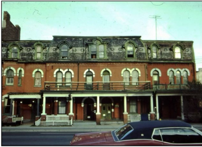
Figure 12. 207-213 Jarvis Street, 1976 (Toronto Historical Board).
