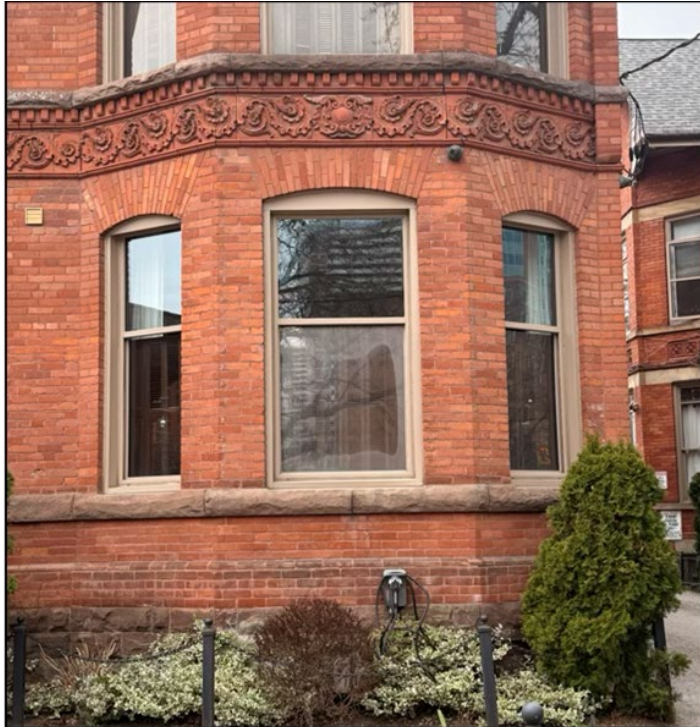
Figure 12. Bay window detail at 506 Jarvis Street showing sandstone foundation sill coursing, and terracotta ornamentation (Alex Corey Heritage Consulting, 2025).
