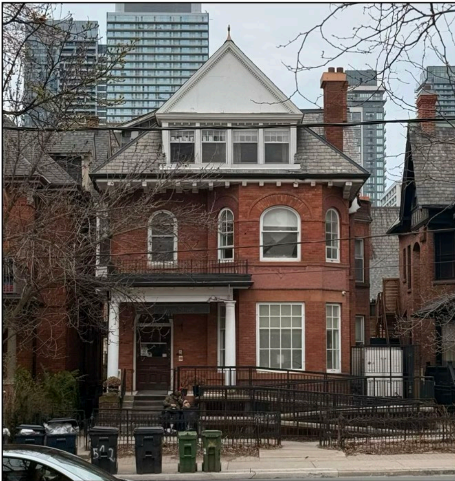
Figure 23. 512 Jarvis Street, primary (west) facade (Alex Corey Heritage Consulting, 2025).
