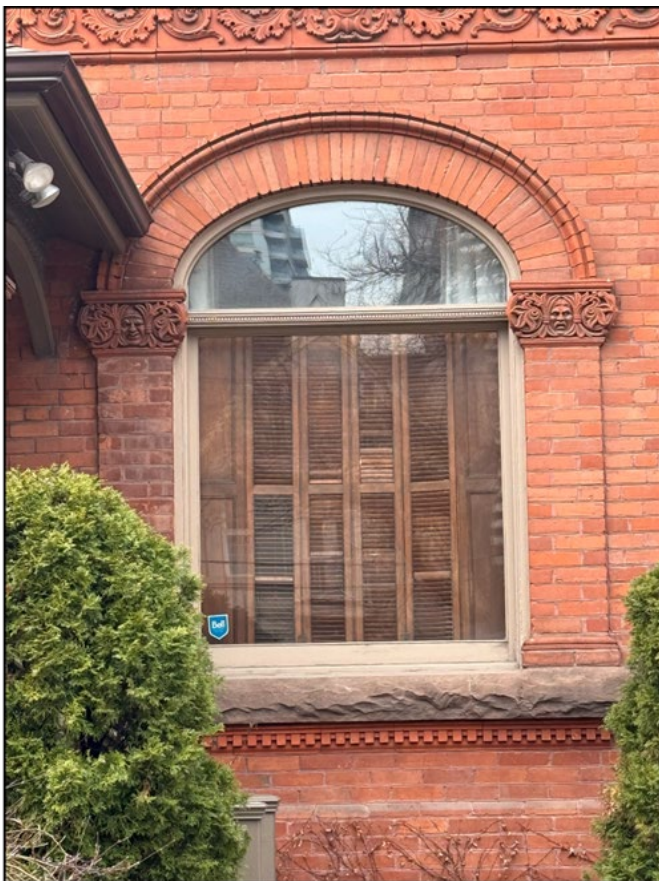
Figure 14. First storey window detail at 506 Jarvis Street showing brick pilasters with terra cotta capitals et beneath a terracotta string course (Alex Corey Heritage Consulting, 2025).
