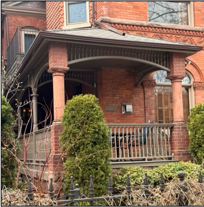
Figure 13. Side porch detail at 506 Jarvis Street showing hipped roof, wood spindles and brick and wood piers and columns (Alex Corey Heritage Consulting, 2025).
