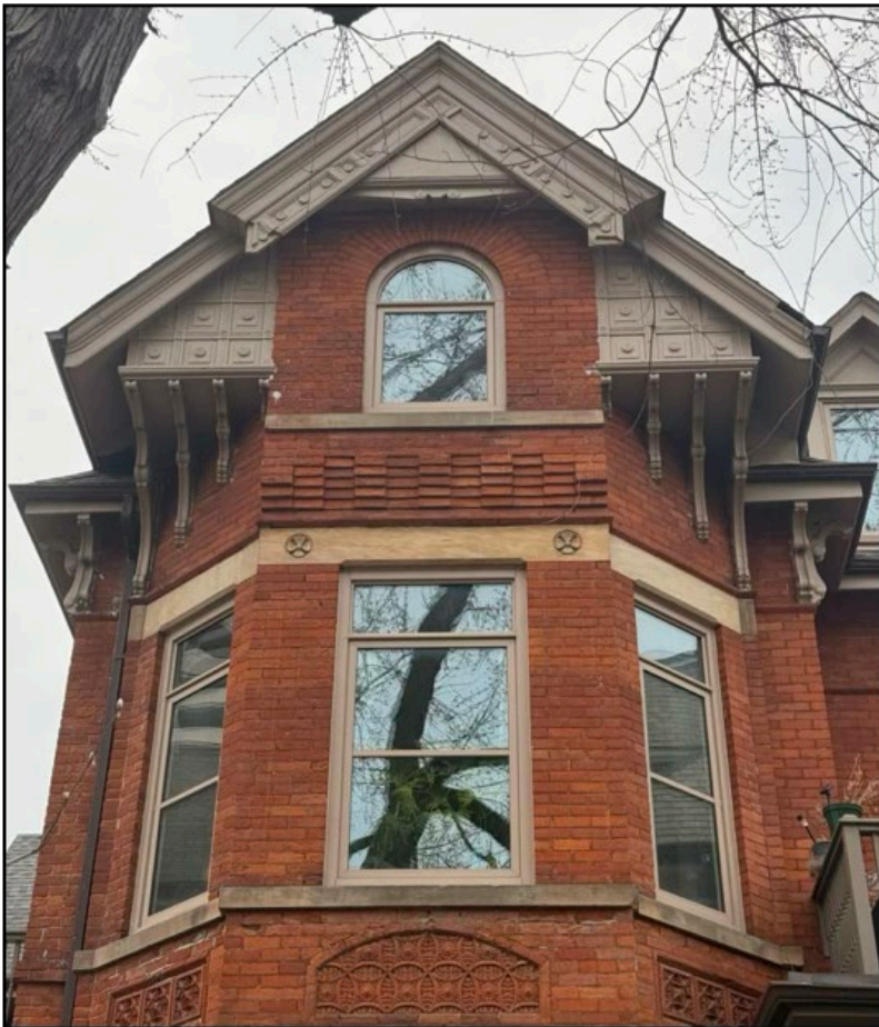
Figure 19. Two-storey bay and gable detail at 510 Jarvis Street showing terracotta panels, sandstone lintels, and wood brackets and bargeboard (Alex Corey Heritage Consulting, 2025).
