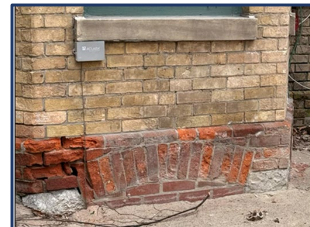
Foundation details at 209 Jarvis Street showing red brick above stone foundation and bricked-in lower-level window opening (Alex Corey Heritage Consulting, 2025).
