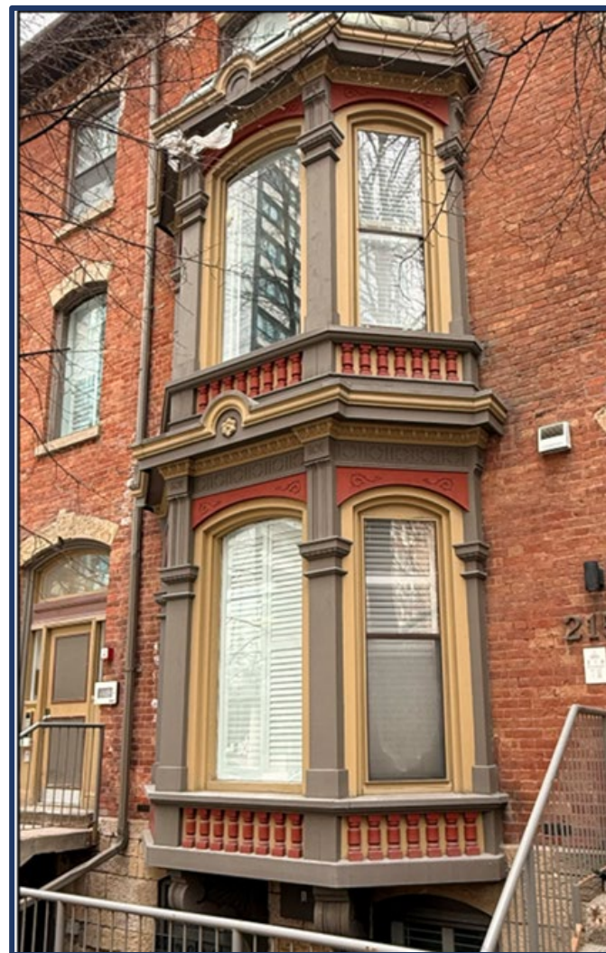
Two-storey bay window detail at 213 Jarvis Street (Alex Corey Heritage Consulting, 2025).
