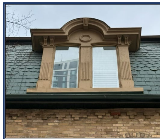
Central double window pedimented dormer detail (Alex Corey Heritage Consulting, 2025).
