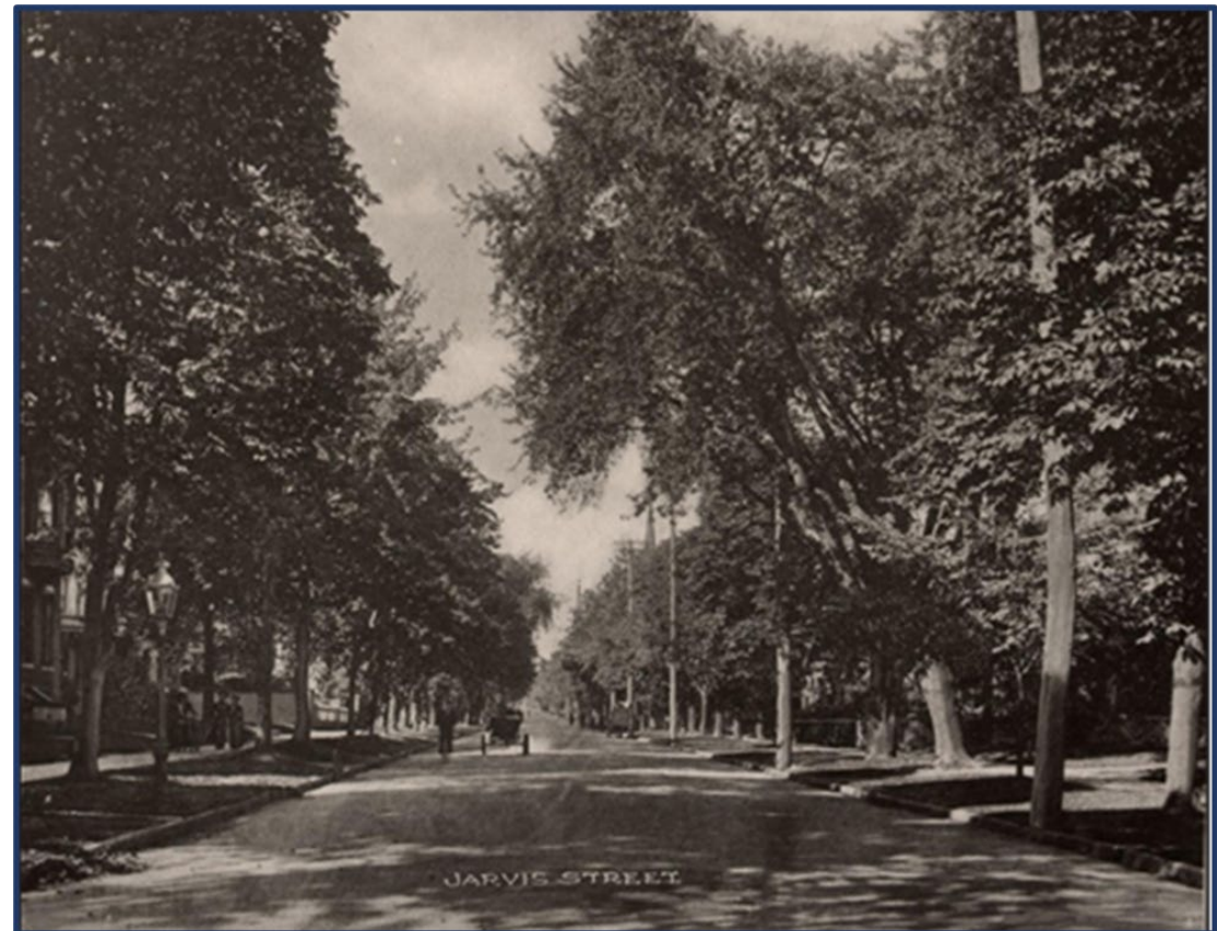
Jarvis Street looking north from about Dundas Street East, 1890 (Toronto Public Library).
