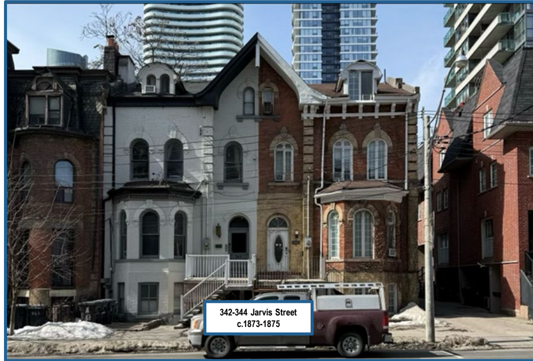
342-344 Jarvis Street (Alex Corey Heritage Consulting, 2025).
