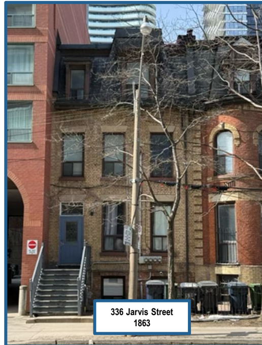
336 Jarvis Street (Alex Corey Heritage Consulting, 2025).
