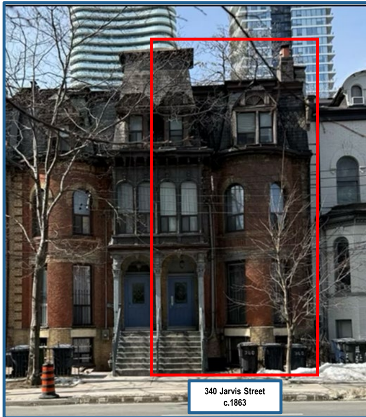
338-340 Jarvis Street (Alex Corey Heritage Consulting, 2025; annotated to show location of subject property).
