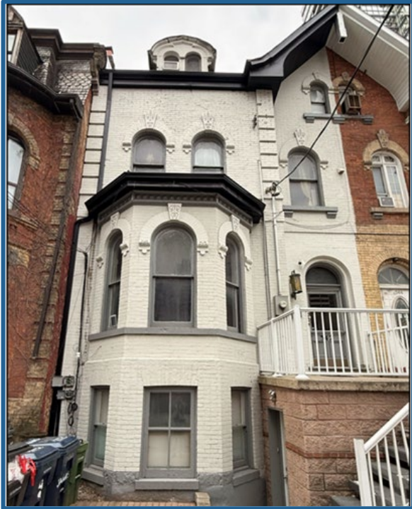
Primary (west) face of 342 Jarvis Street showing ornamentation that has been painted over (Alex Corey Heritage Consulting, 2025).
