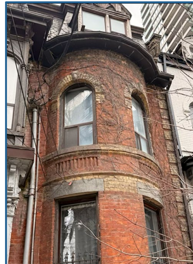
Two-storey bay window detail at 340 Jarvis Street (Alex Corey Heritage Consulting, 2025).
