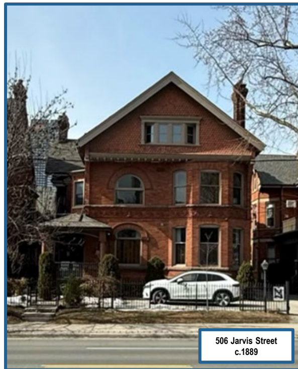
506 Jarvis Street (Alex Corey Heritage Consulting, 2025).
