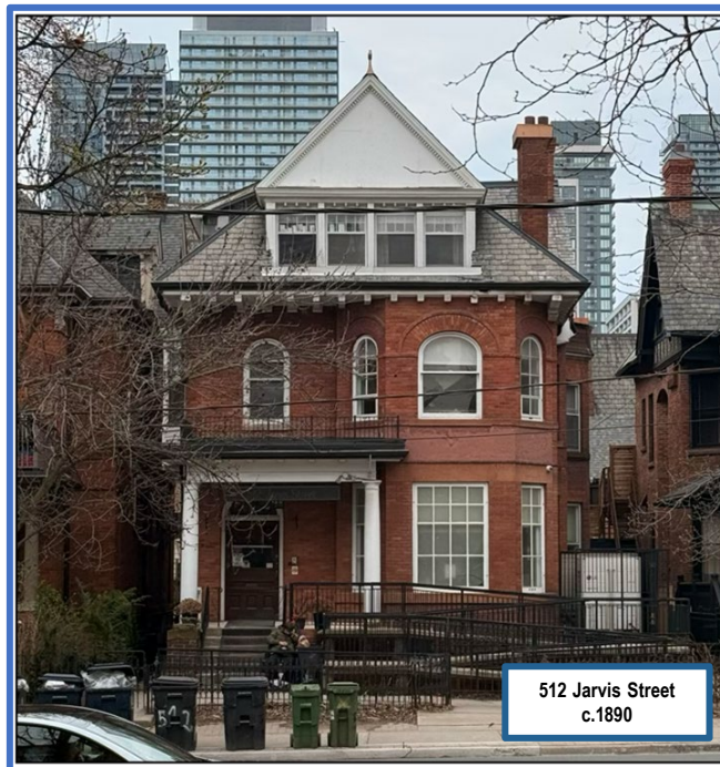
512 Jarvis Street, primary (west) facade (Alex Corey Heritage Consulting, 2025).
