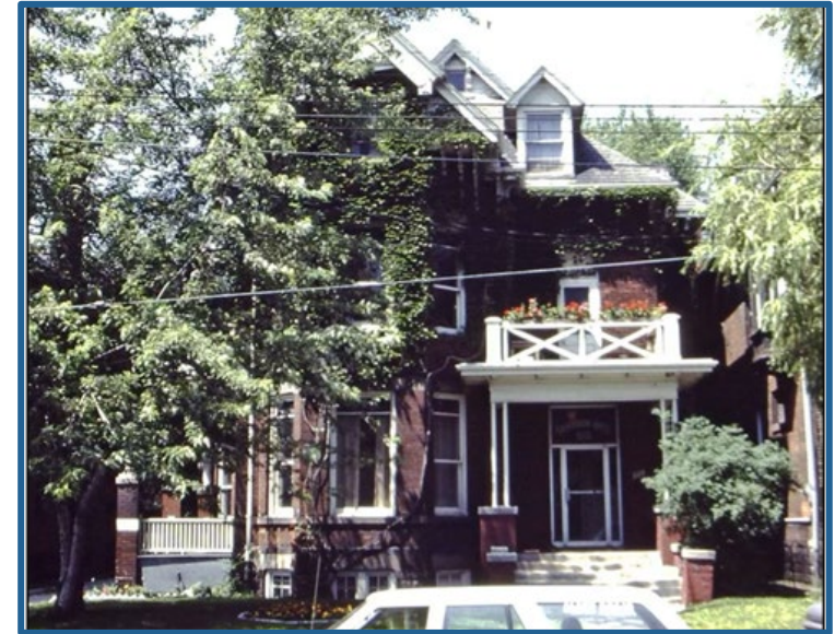
510 Jarvis Street, 1980 (Toronto Historical Board).
