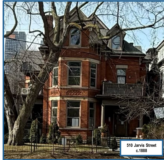
510 Jarvis Street (Alex Corey Heritage Consulting, 2025).
