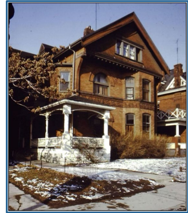
506 Jarvis Street, 1976 (Toronto Historical Board).
