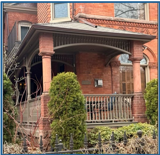
Side porch detail at 506 Jarvis Street showing hipped roof, wood spindles and brick and wood piers and columns (Alex Corey Heritage Consulting, 2025).
