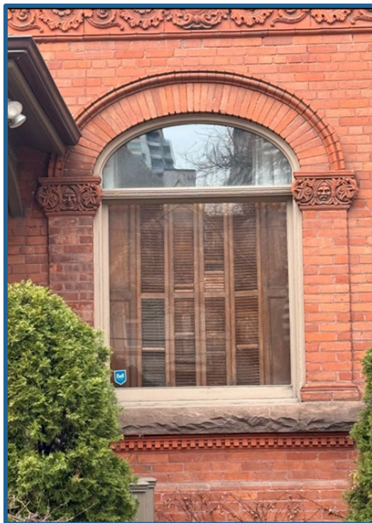
First storey window detail at 506 Jarvis Street showing brick pilasters with terra cotta capitals and beneath a terracotta string course (Alex Corey Heritage Consulting, 2025).
