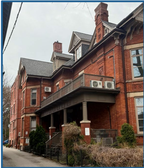
Secondary (south) facade of 510 Jarvis Street with apartment addition at rear (Alex Corey Heritage Consulting, 2025).
