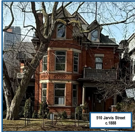
510 Jarvis Street (Alex Corey Heritage Consulting, 2025).
