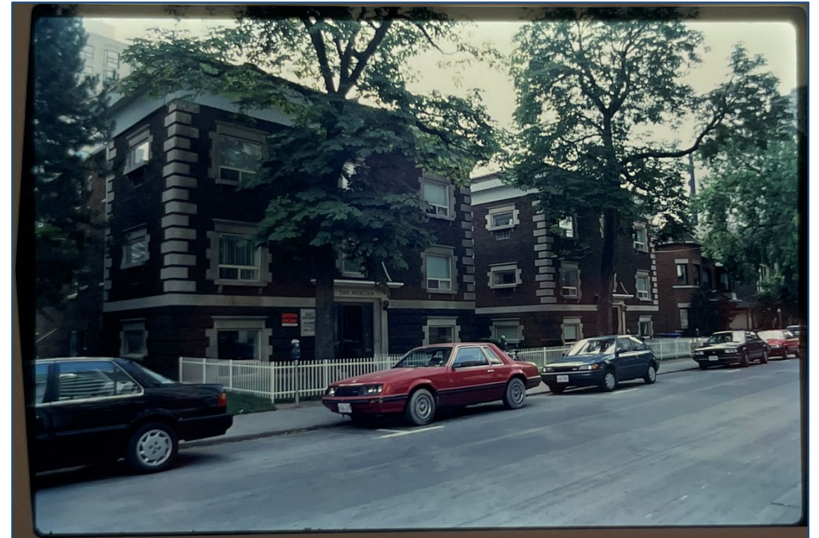
1992 photograph of 81 Isabella Street, cornice and brick parapet have been over-clad (CTA).
