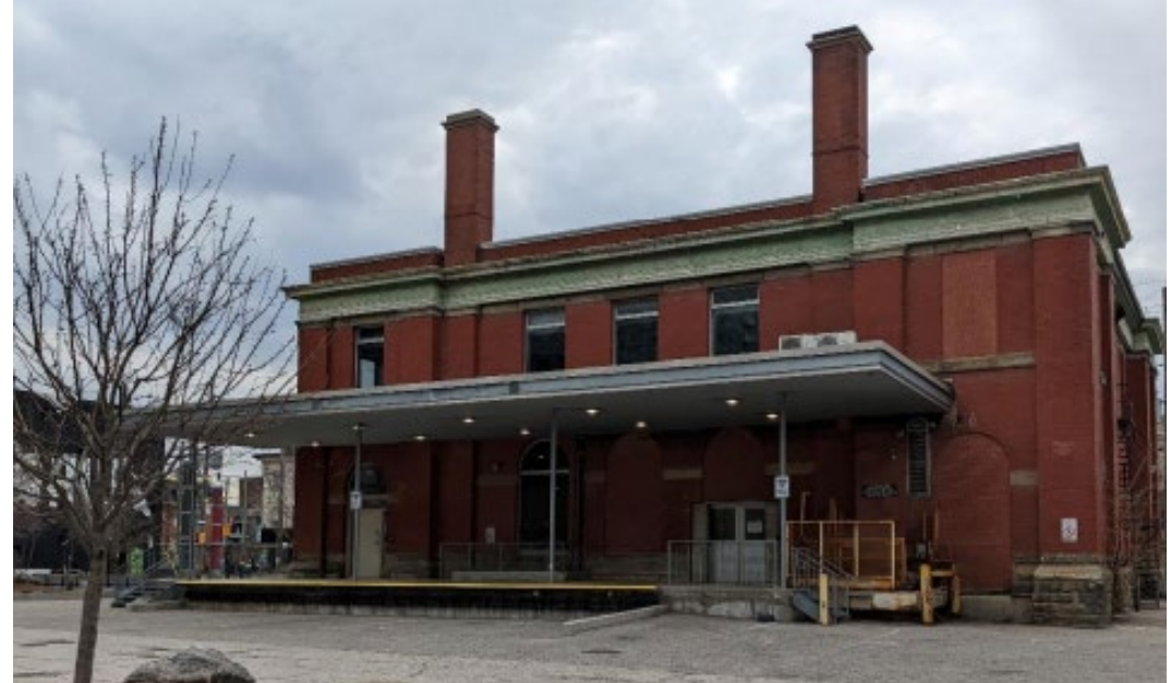
Rear (south) Elevation fronting Lisgar Park
