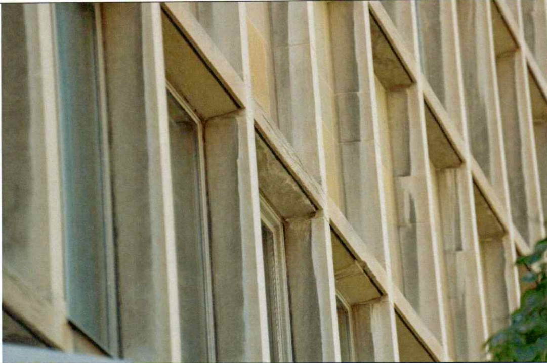
Figure 80 West elevation eroded lintel stone and area of damaged drip edge at the 5 th -floor windows.
