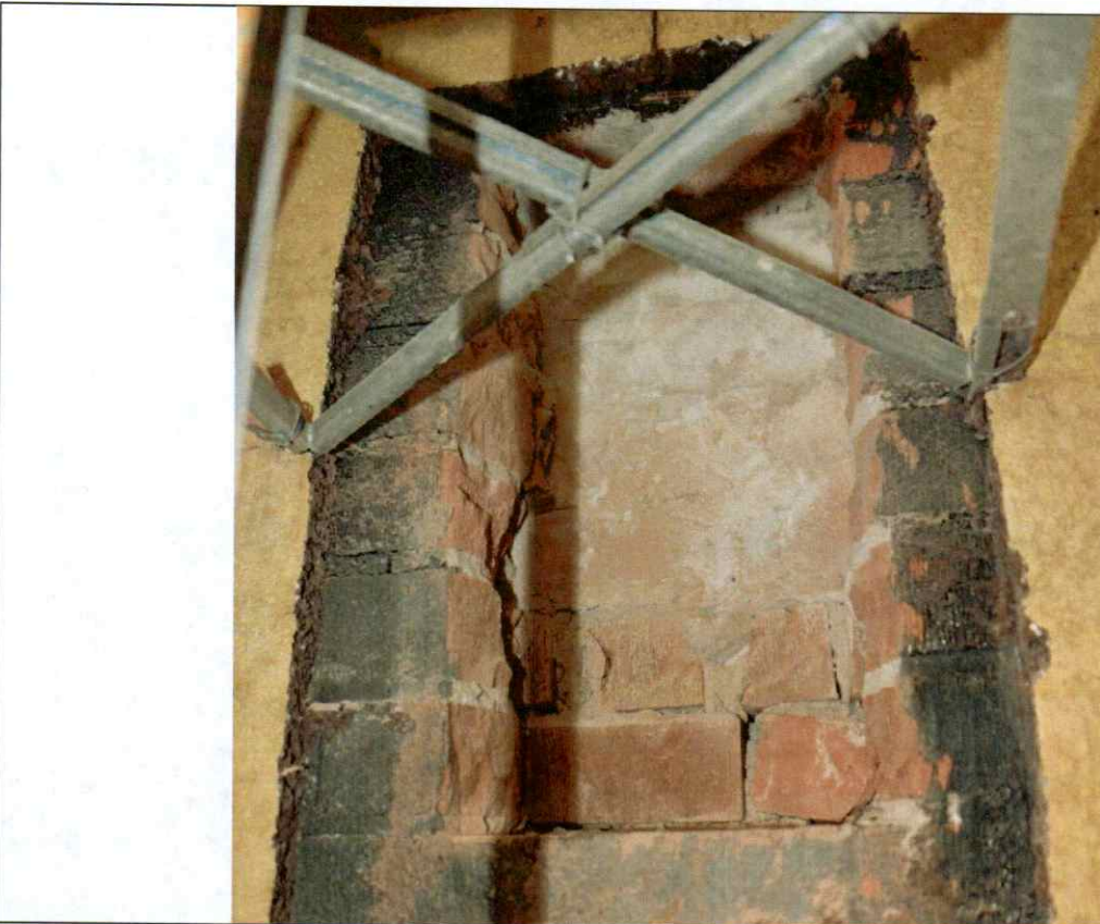
Figure 47 Investigation opening #19 Detail. Corkboard and brick masonry were removed. Stone is block bonded into backup.
