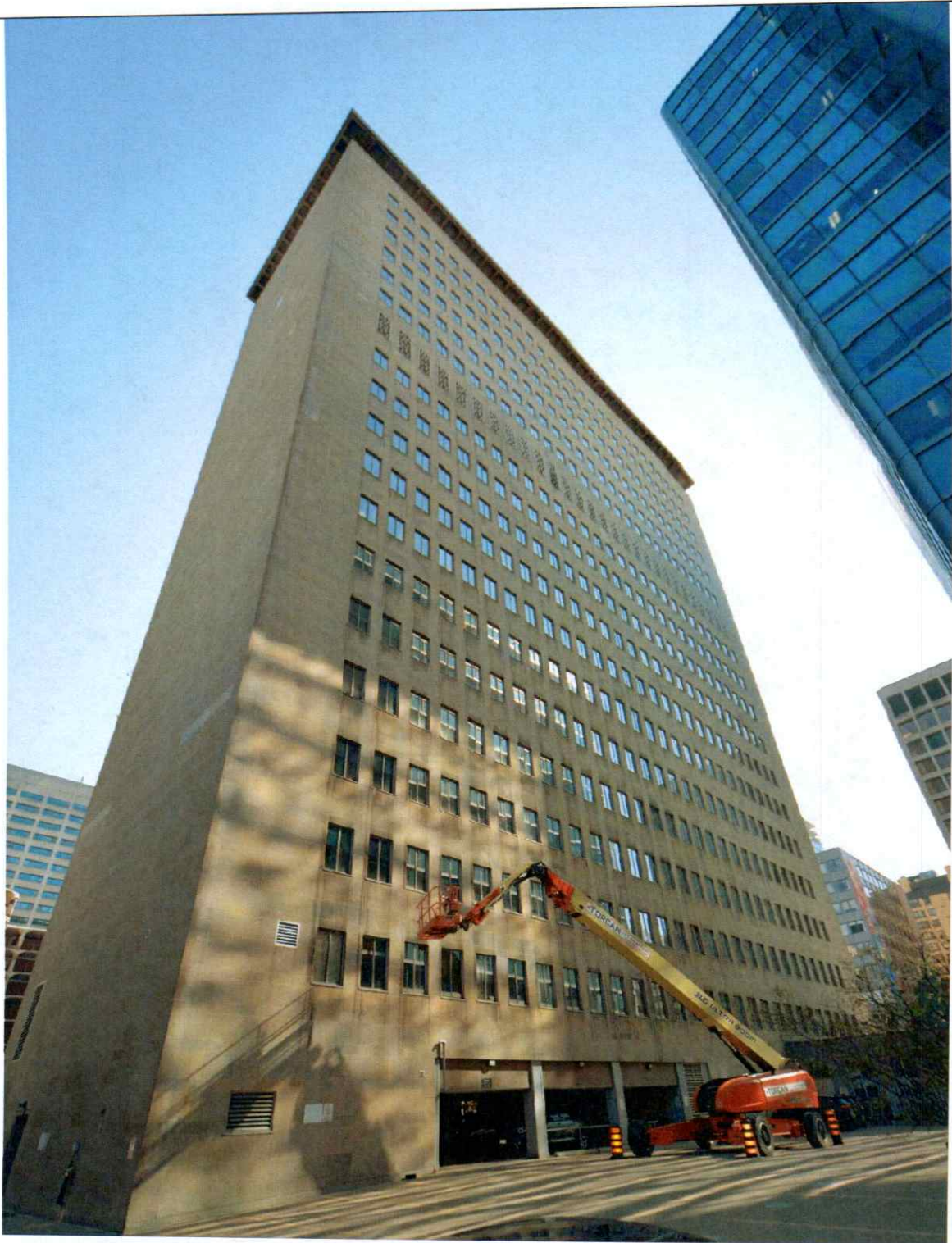
Figure 8 Overview of the north elevation.
