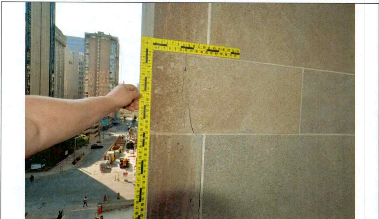
Figure 73 North elevation northeast corner. Detail of Crack/ displacement at 3 rd floor.
