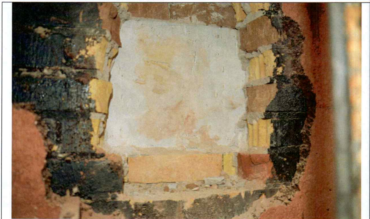
Figure 37 Investigation opening #14 Detail. Corkboard and brick masonry were removed. Stone is block bonded into backup.
