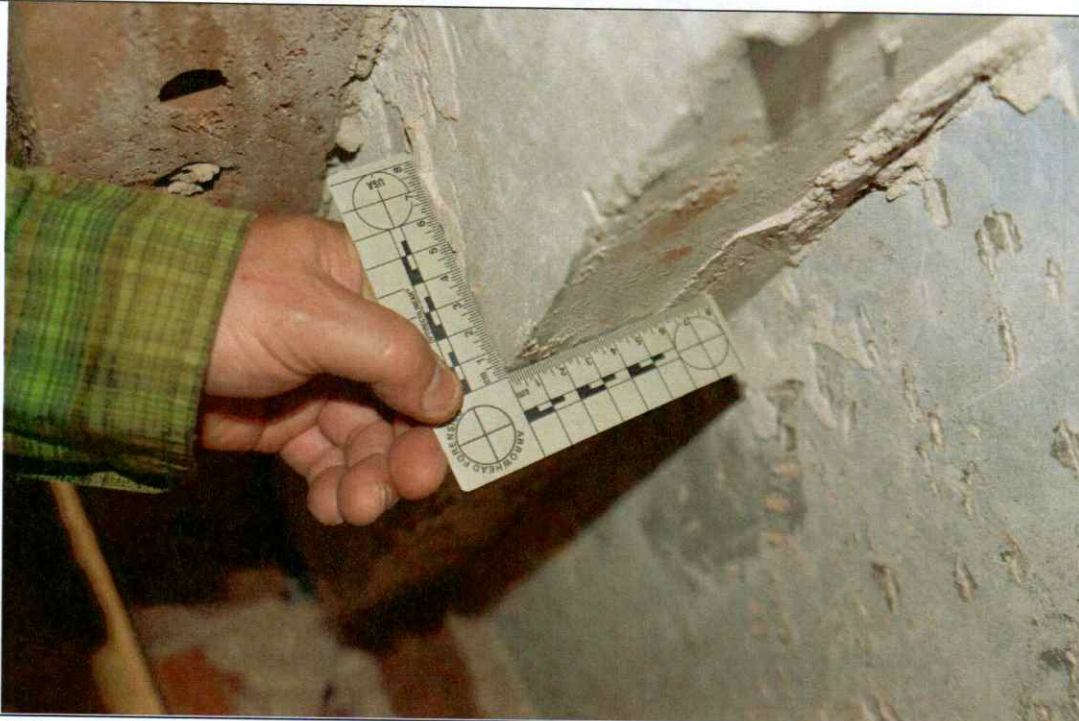
Figure 19 Investigation opening #5 Detail. Stone veneer is block bonded with brick backup. No ties were found.
