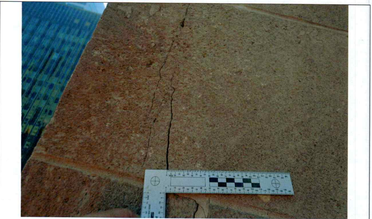
Figure 71 North elevation northeast corner. Detail of Crack/ displacement at 3 rd floor.
