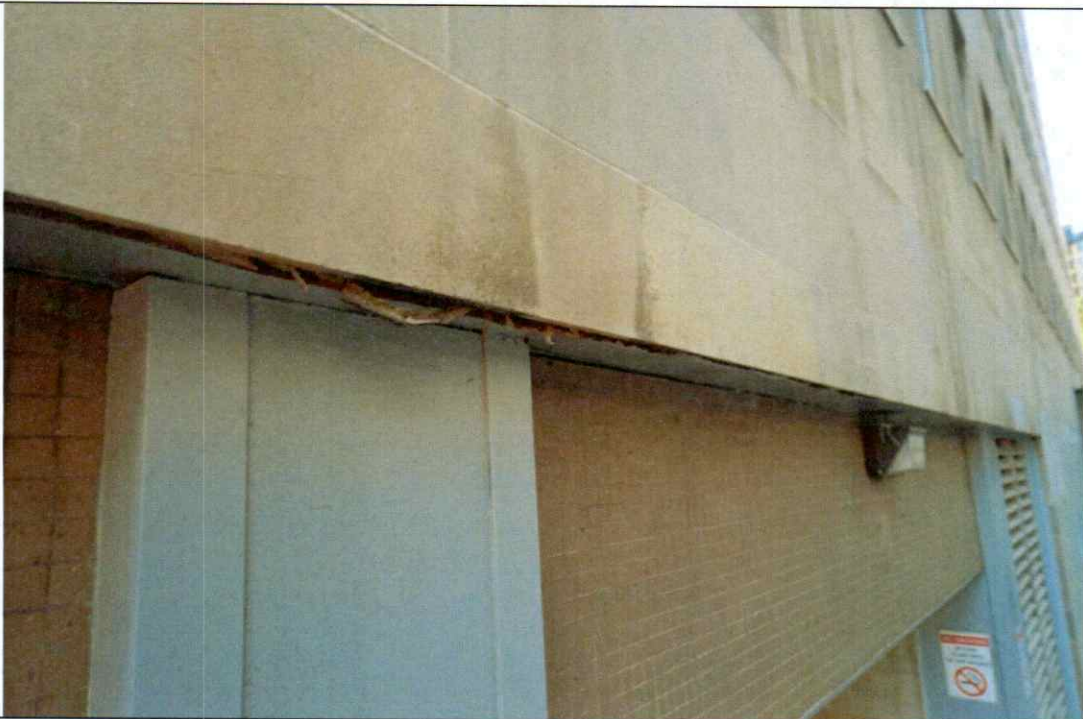
Figure 77 North elevation first-floor soffit sealant has failed and there is some evidence of internal corrosion of steel elements (rusting and some displacement at the soffit plate) along this elevation.
