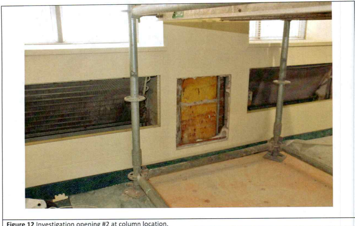
Figure 12 Investigation opening #2 at column location.
