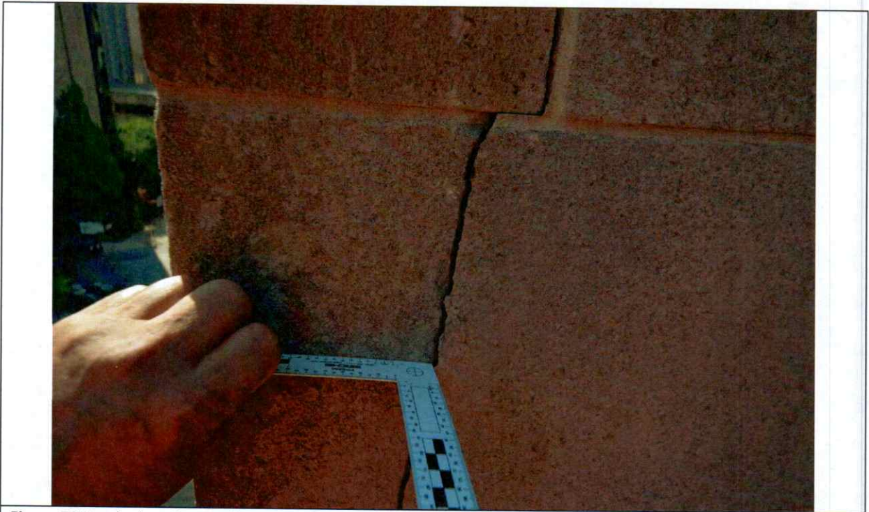
Figure 70 North elevation northeast corner. Detail of Crack/ displacement at 4 th floor.
