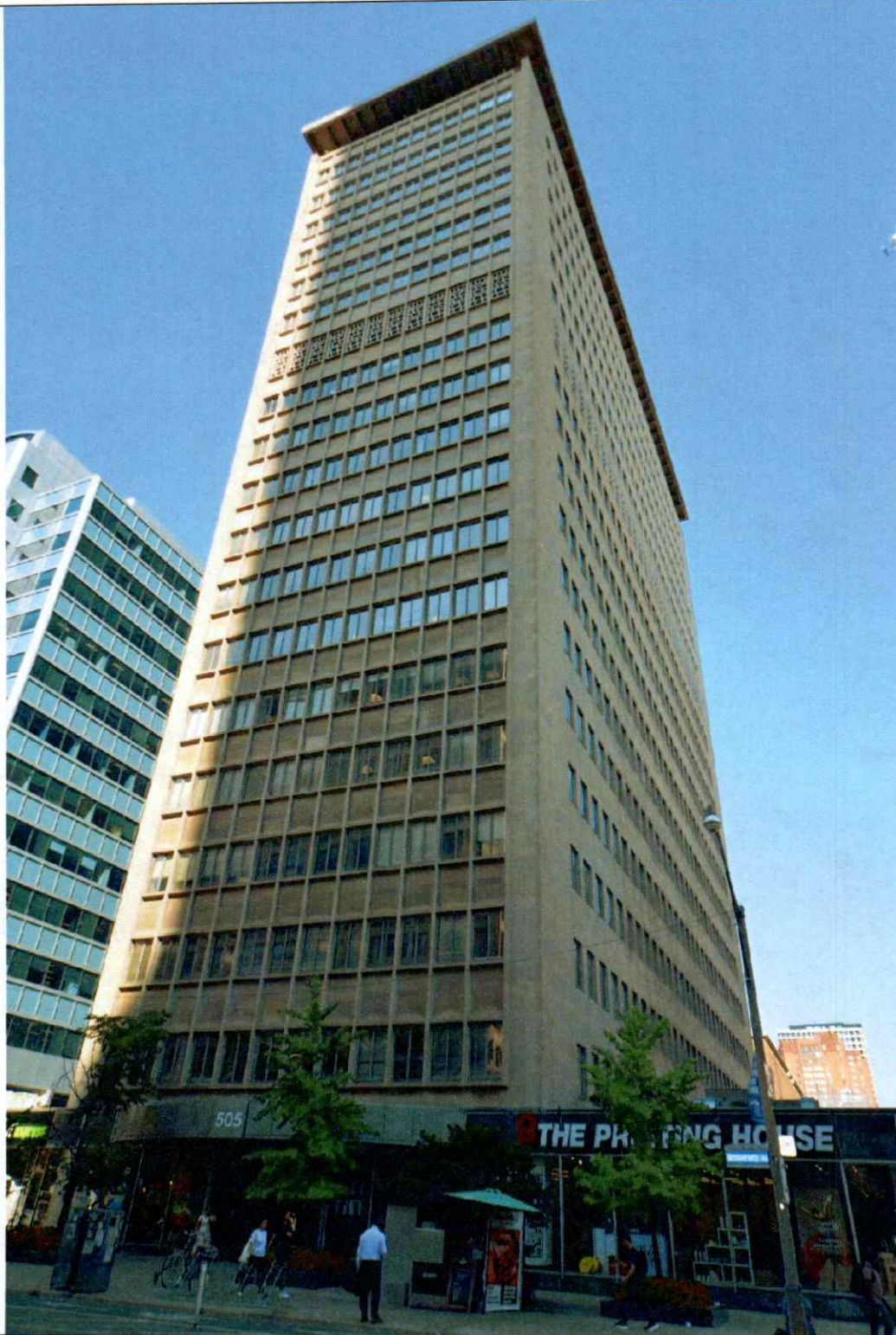
Figure 9 Overview of the west elevation.
