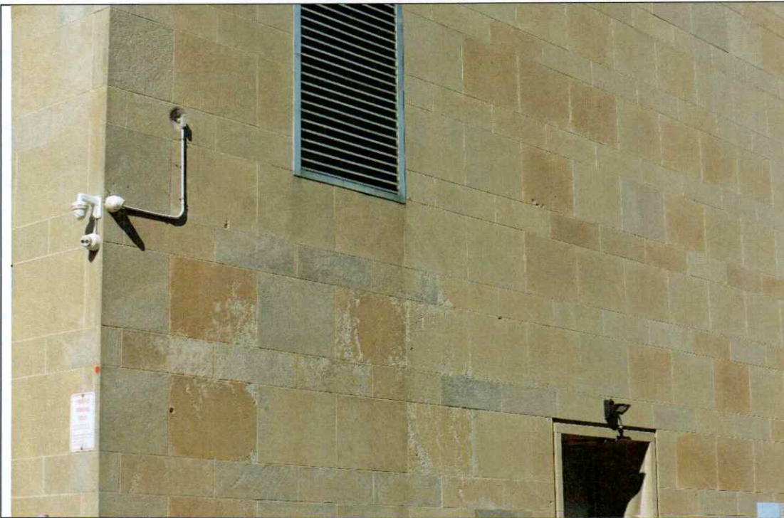
Figure 65 East elevation ground to 2 nd floor. Surface erosion/ exfoliation related to moisture from the vent above.
