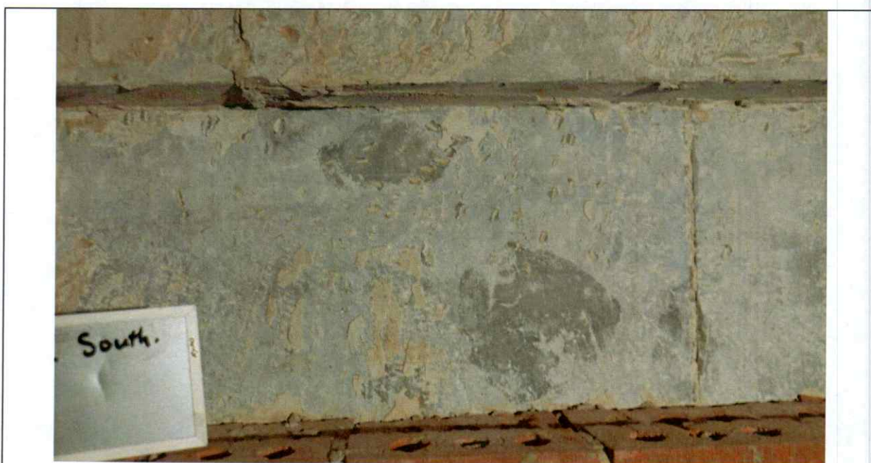
Figure 11 Investigation opening #1 Detail. Stone veneer is block bonded with brick backup. No ties were found here.
