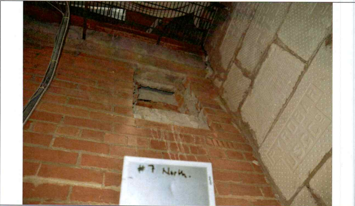
Figure 22 Investigation opening #7 in vent shaft underside of the ring beam.
