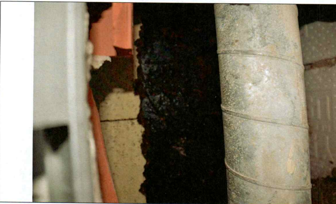
Figure 27 Investigation opening #9 Detail. The corkboard insulation was removed. A bituminous layer over parged stone masonry was found.
