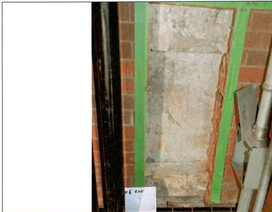
Figure 21 Investigation opening #6 Detail. Stone veneer is block bonded with brick backup. No ties were found.
