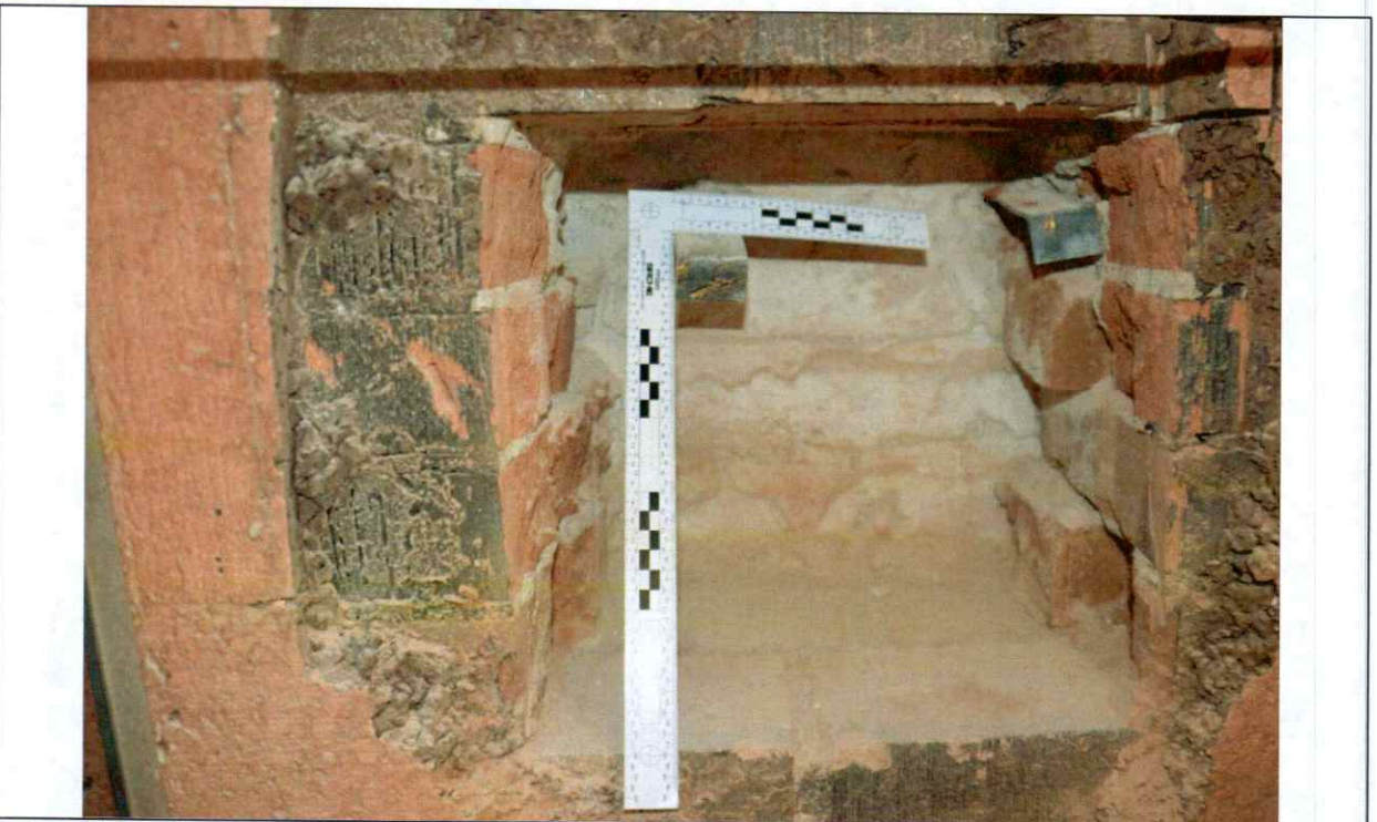
Figure 39 Investigation opening #15 Detail. Corkboard and brick masonry were removed. 2 ties were found- ties appear to be bronze (or similar copper alloy) and in good condition.
