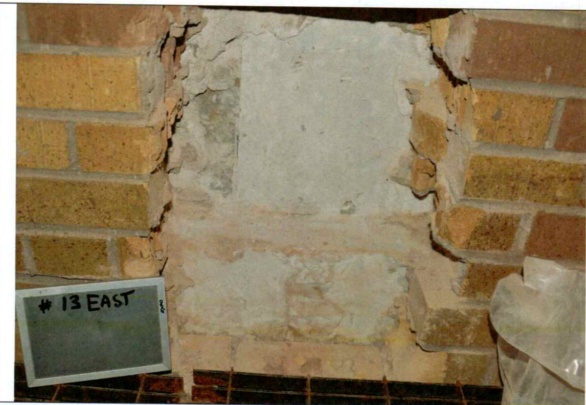
Figure 35 Investigation opening #13 in vent shaft Detail. Stone veneer is block bonded with brick backup. No ties were found.
