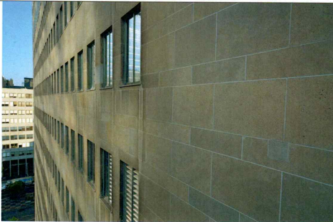
Figure 55 South elevation at the 5 th floor. The masonry is in good condition. Note replaced window mullion panel- Indiana limestone and surface mortar patch (RHS).
