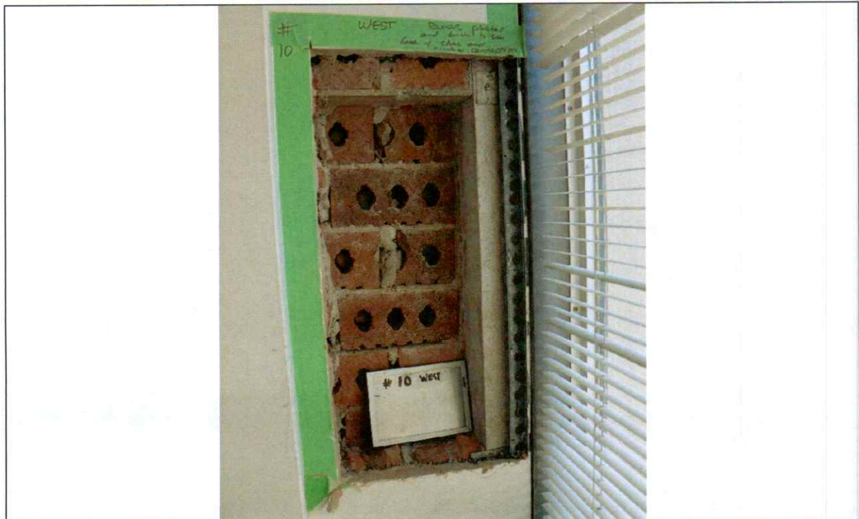
Figure 28 Investigation opening #10 window mullion.
