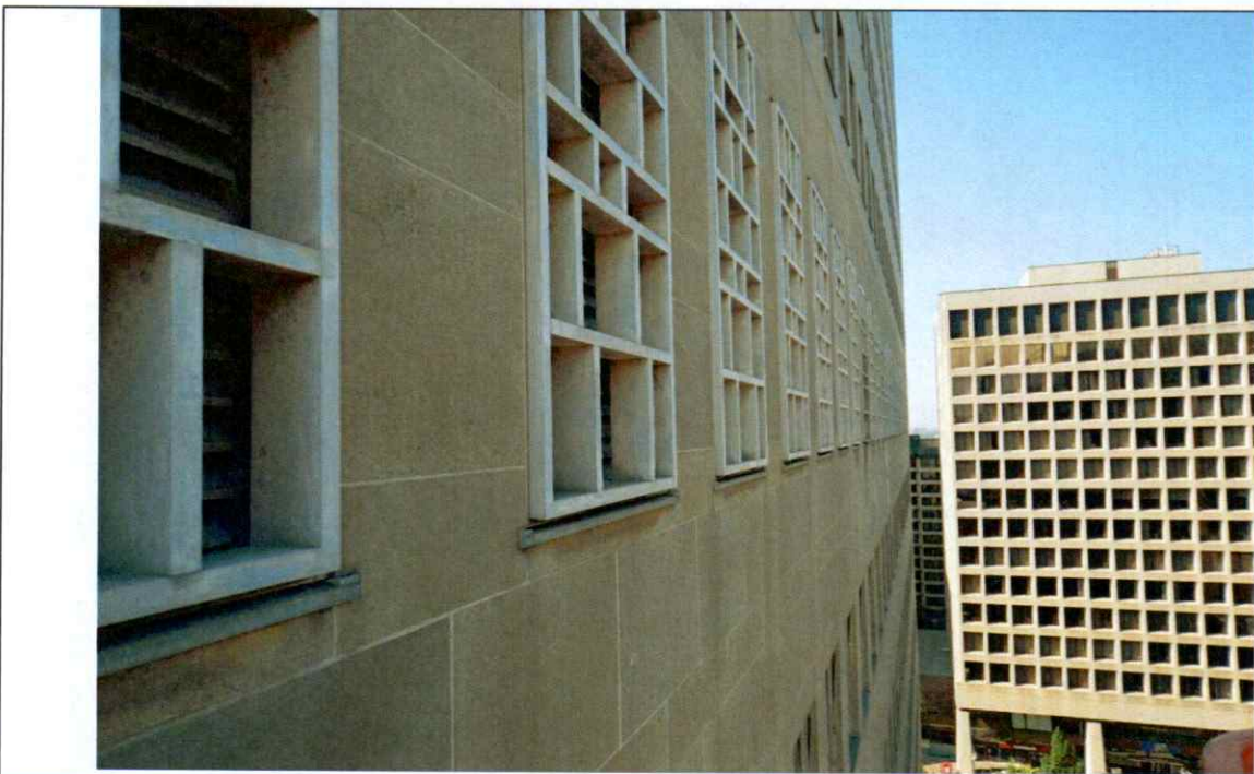
Figure 75 North elevation vent screens at the 13 th floor. The masonry is generally in good condition.
