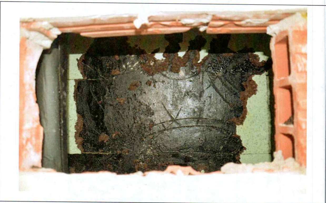
Figure 51 Investigation opening #21 Detail. The corkboard was removed back of the stone was parged and bitumen paint coated.
