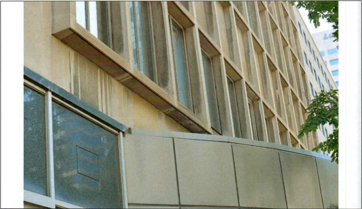
Figure 78 West elevation eroded sill at the 2 nd floor window.
