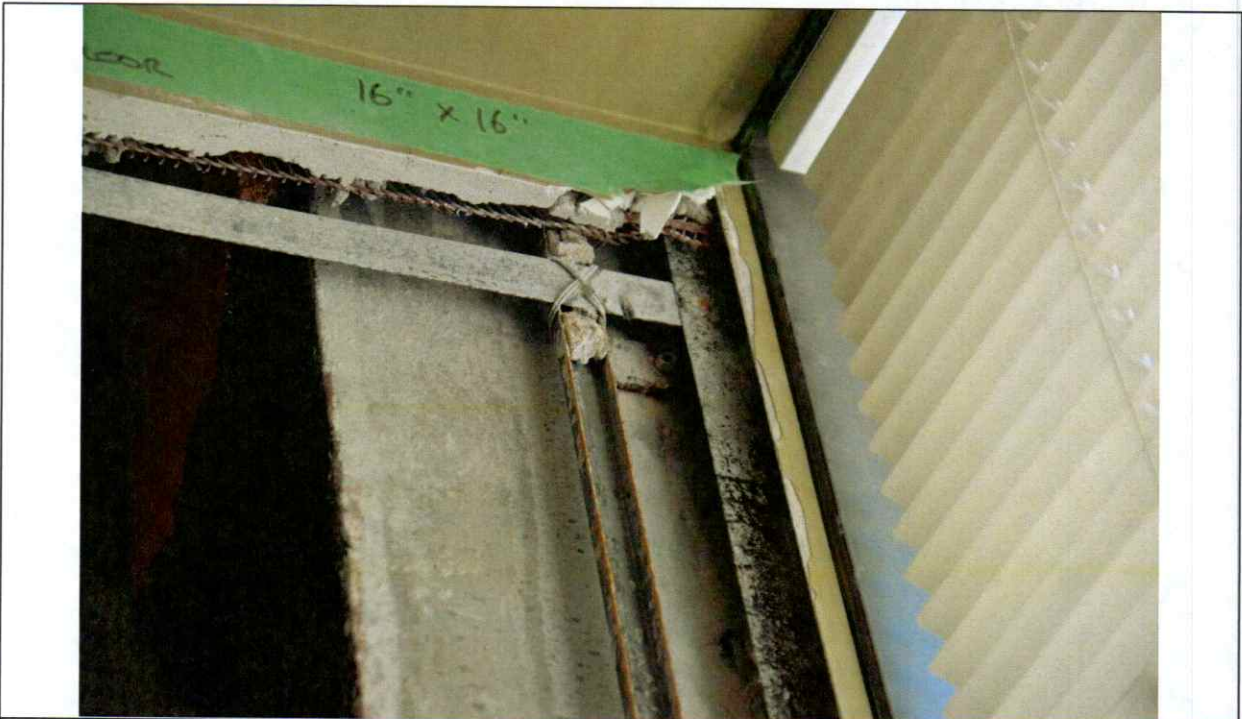
Figure 43 Investigation opening #17 Detail. Mullion stone is full depth- no backup masonry is present. Some light corrosion is evident on plaster framing elements. Window ties are anchored with #12 Galvanized screws into stone.
