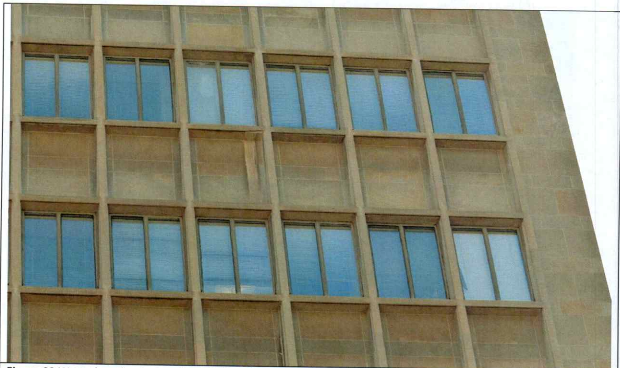
Figure 83 West elevation lost section of drip edge on the sill at the 9 th floor.
