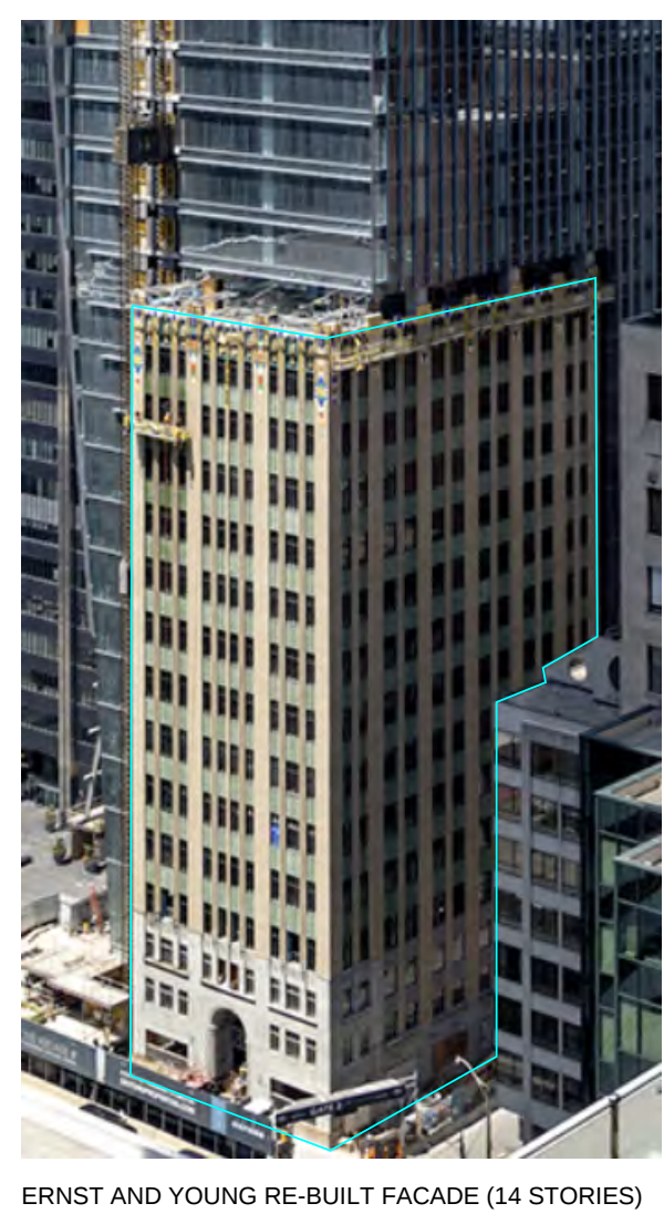
ERNST AND YOUNG RE-BUILT FACADE (14 STORIES)
