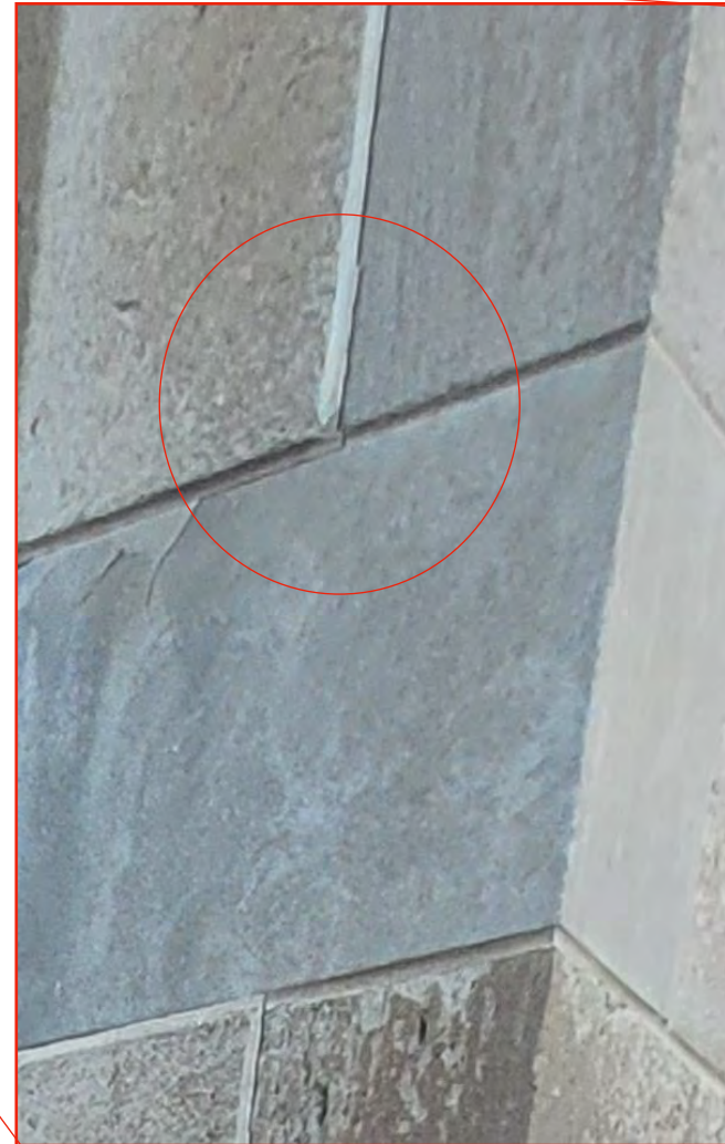
Cracking at southeast corner (4 th Floor extending to grade). Joint repairs within the past 20 years are again opening up (circle in the magnified detail. Similar conditions occur at other corners (particularly the northeast and southwest although the base of the building at the west is partially constrained by the podium causing less damage at the west corners).
