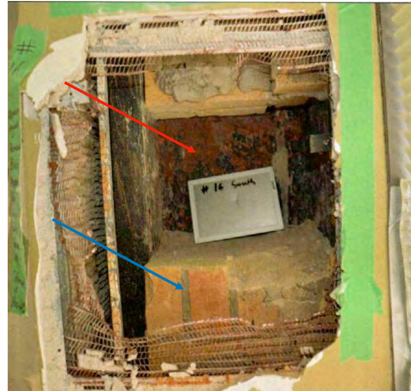
Illustration from the Clifford Restoration report. The red arrow points to the web of a steel H column into which masonry (blue arrow) has been built. The masonry is built tight to the flanges and web of the column. The steel is corroding at this middle level floor – lower floors will see greater levels of corrosion due to ponding of water.
