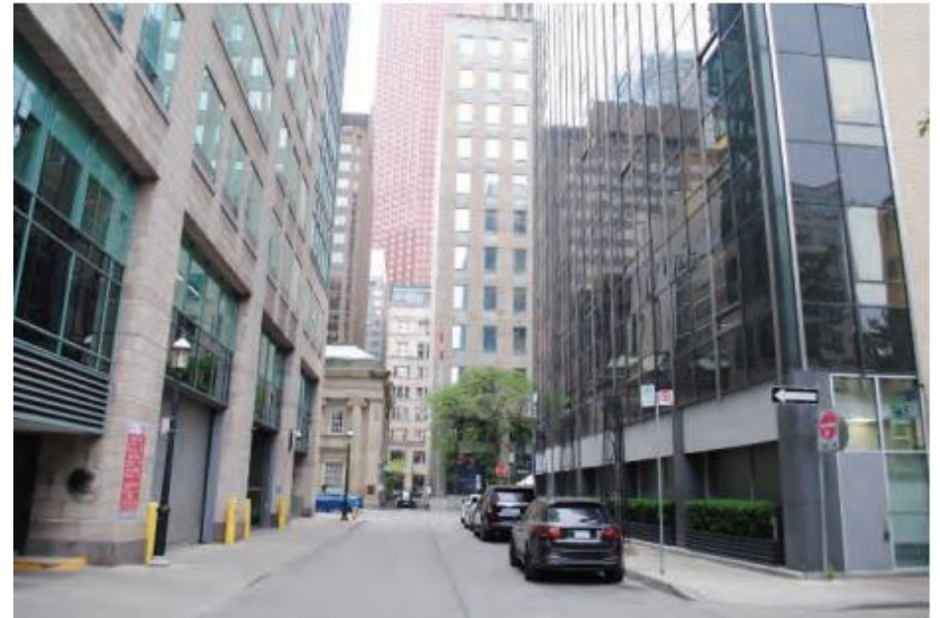
South (side) and East (rear) elevations of 15 Toronto Street looking west (GBCA Architects Ltd., 2023).
