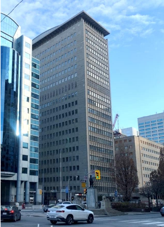
West and North Elevations
