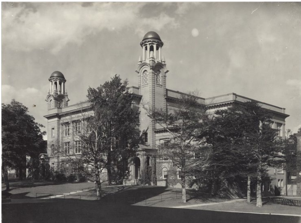
Figure 3: The Medical School Building, view from southwest; the building was designed by Darling and Pearson and constructed 1903. Photograph c.1922 (University of Toronto Archives).
