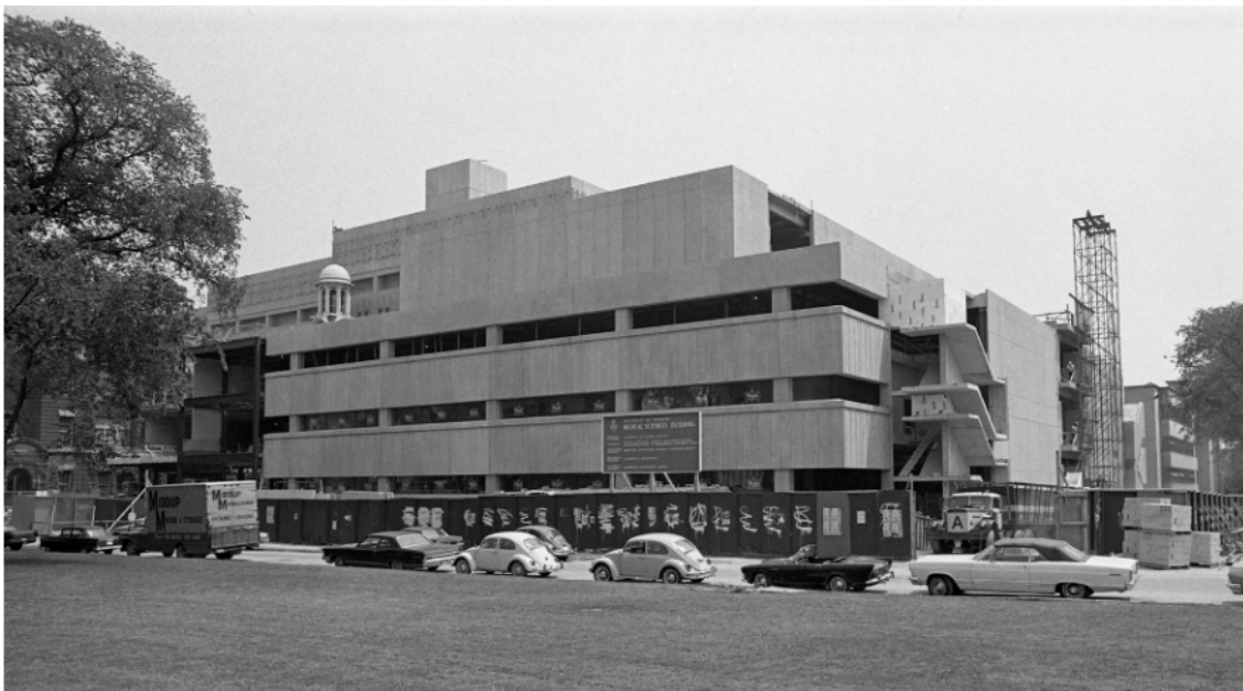
Figure 4: The Medical Sciences Building during construction, prior to the demolition of the old Medical School Building, which is visible towards the left of the image. (University of Toronto Archives).
