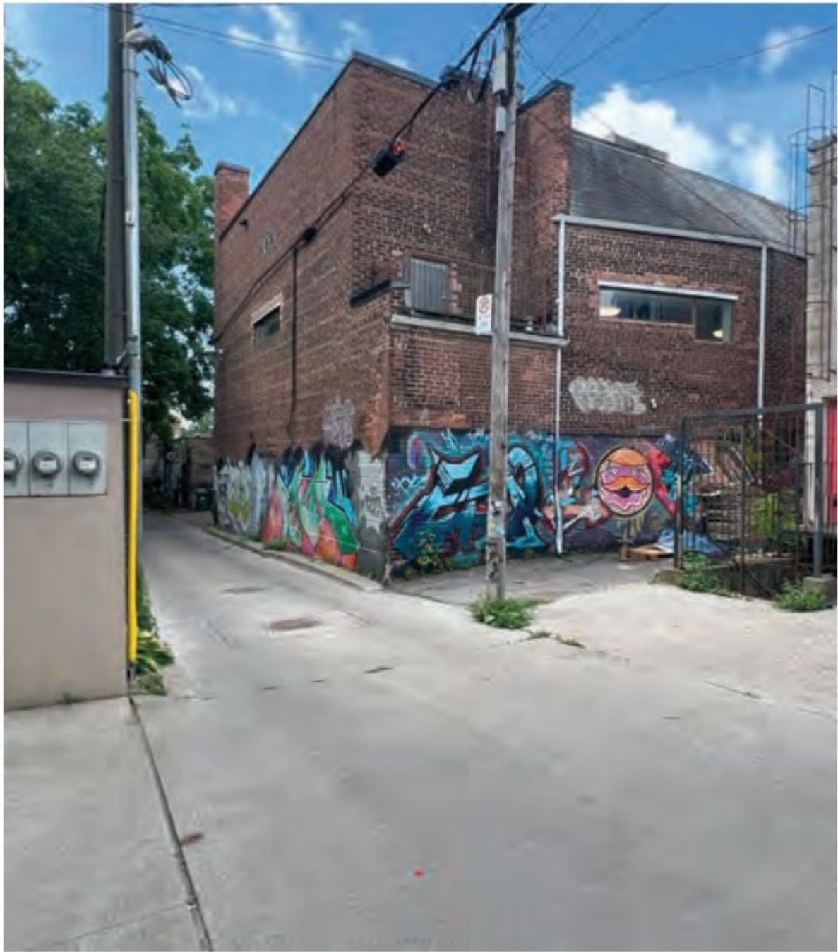
Figure 5. East elevation of 509 Parliament Street, looking southwest (ERA Architects Inc., 2025).
