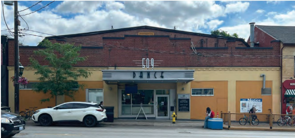
Figure 3. Principal (west) elevation of 509 Parliament Street (ERA Architects Inc., 2025).
