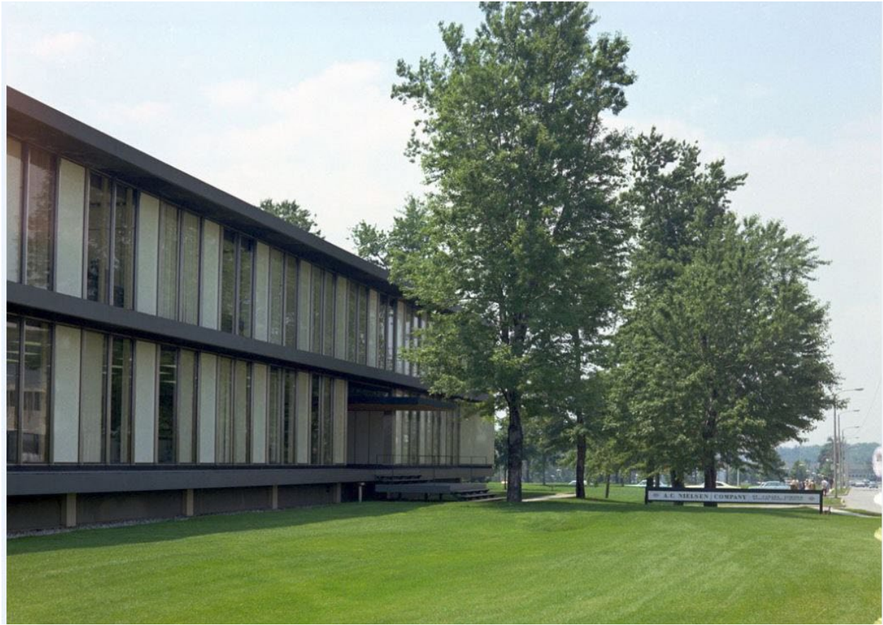
Figure 3 1960s image looking west showing the Principal (north) elevation of 39 Wynford Drive prior to the addition of 2 storeys in 1967 (Toronto Archives).
