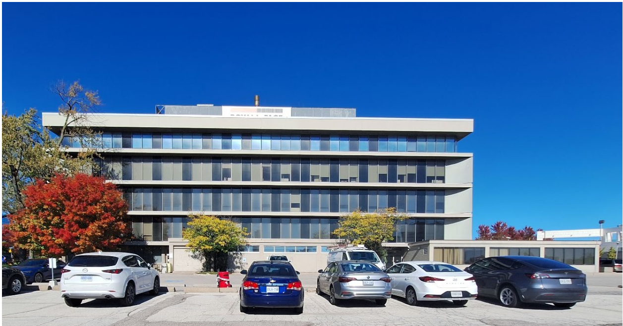
Figure 10 South (rear) elevation of 39 Wynford Drive. Note 1-storey basement additions at the centre and right (Heritage Planning, 2025).
