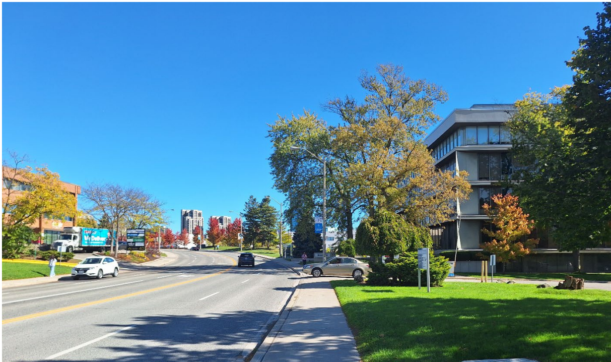
Figure 14 View looking east from the intersection of Wynford Drive and Gervais Drive with 39 Wynford Drive on the right (Heritage Planning, 2025).
