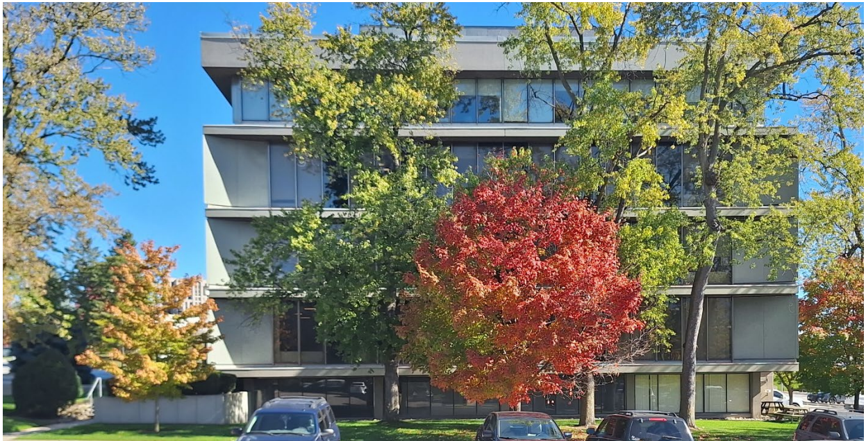
Figure 9 West elevation of 39 Wynford Drive (Heritage Planning, 2025).
