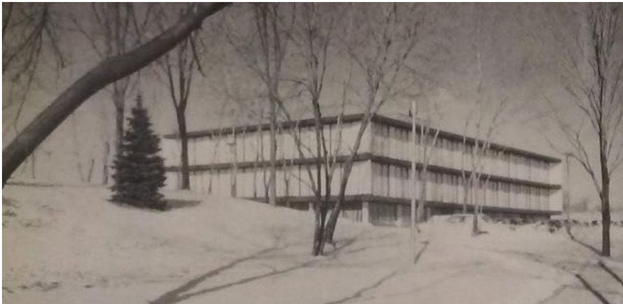
Figure 2 Image looking northeast from Gervais Drive showing, left to right, the west and rear (south) showing the original 2-storey structure with walk out basement (ASI, 2019; The Canadian Architect 1963:58).
