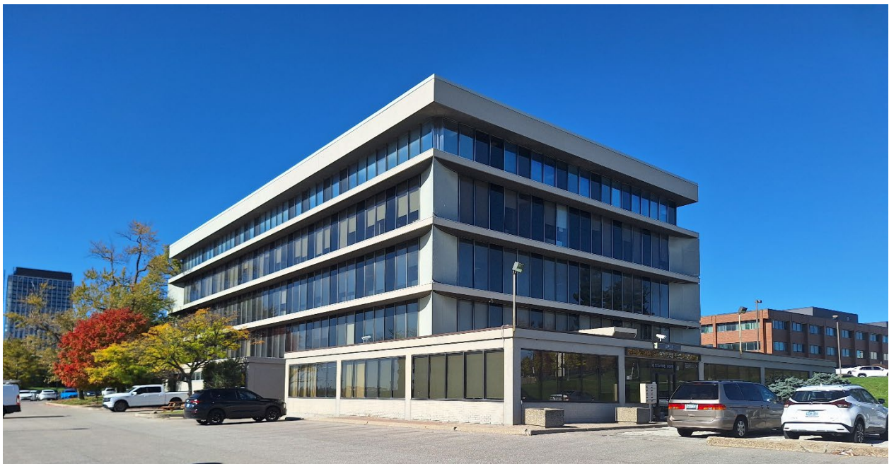
Figure 11 Northwest view of rear and west east elevations showing curved corner walls and basement additions (Heritage Planning, 2025).
