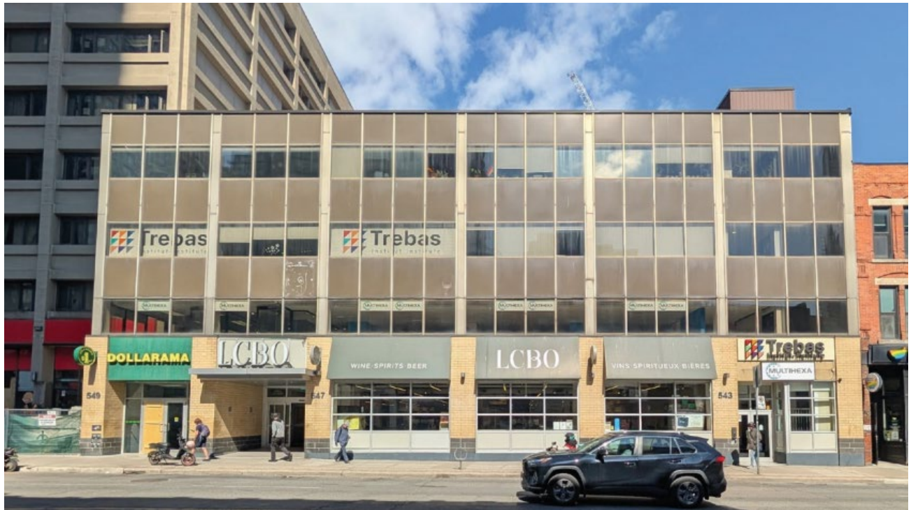
West (principal) elevations at Yonge Street frontage of 543 Yonge Street ERA Architects)
