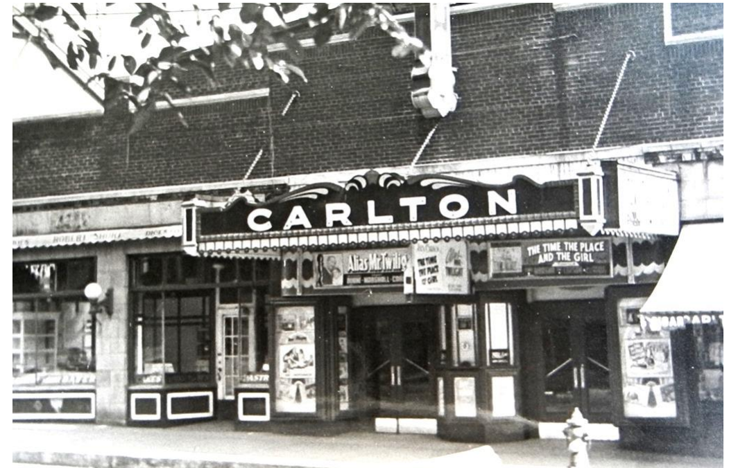
Pre-1940 photograph of the principal (west) elevation of 509 Parliament Street (City of Toronto Archives).
