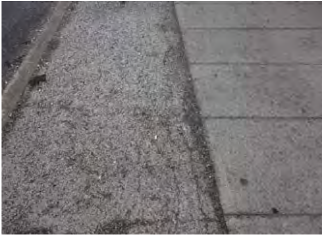
Plate 151: Concrete sidewalk with porous concrete border
