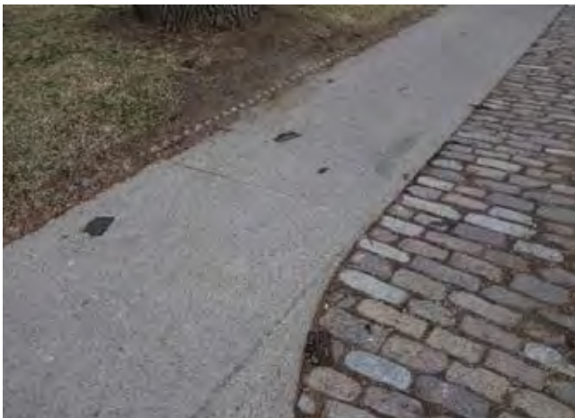
Plate 149: Concrete sidewalk with granite setts
