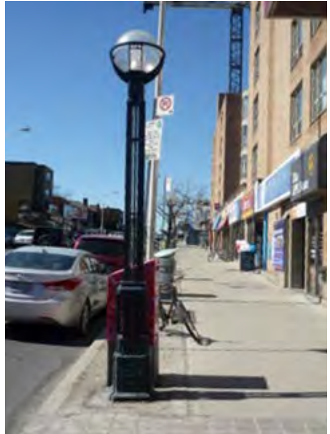
Plate 148: Type II pedestrian light with steel pole and base cover in the Study Area
