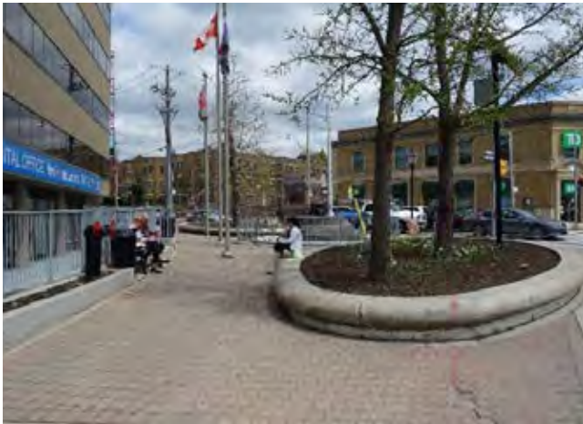
Plate 153: : Interlocking stone plaza and decorative concrete seat wall planter with trees
