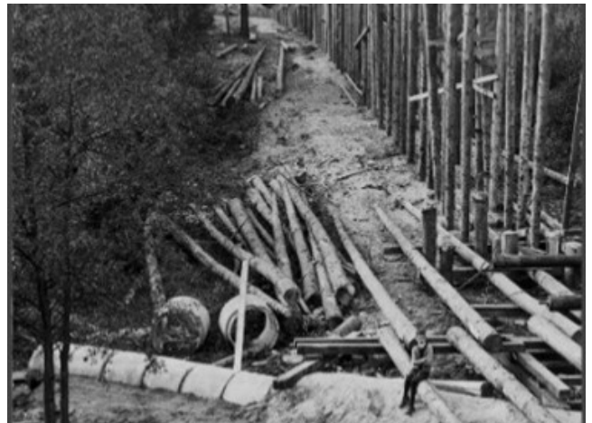
Plate 24: Bloor Street West at High Park Piles for Bridge, 1914 (Source: City of Toronto Archives 1914c)
