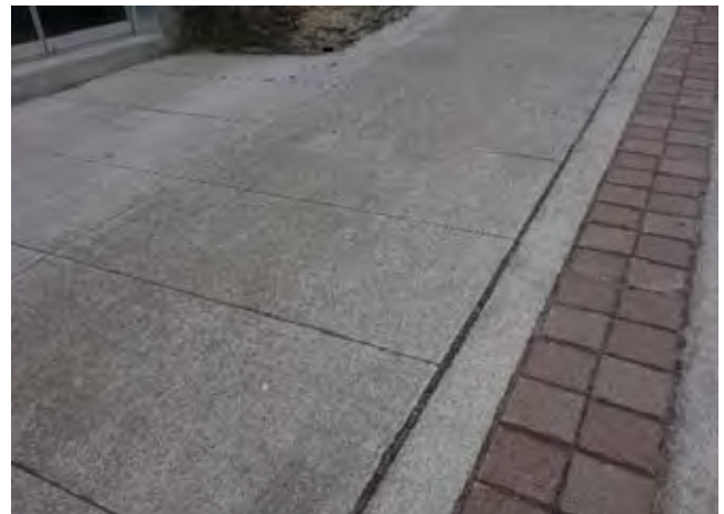
Plate 150: Concrete sidewalk with concrete unit paver band
