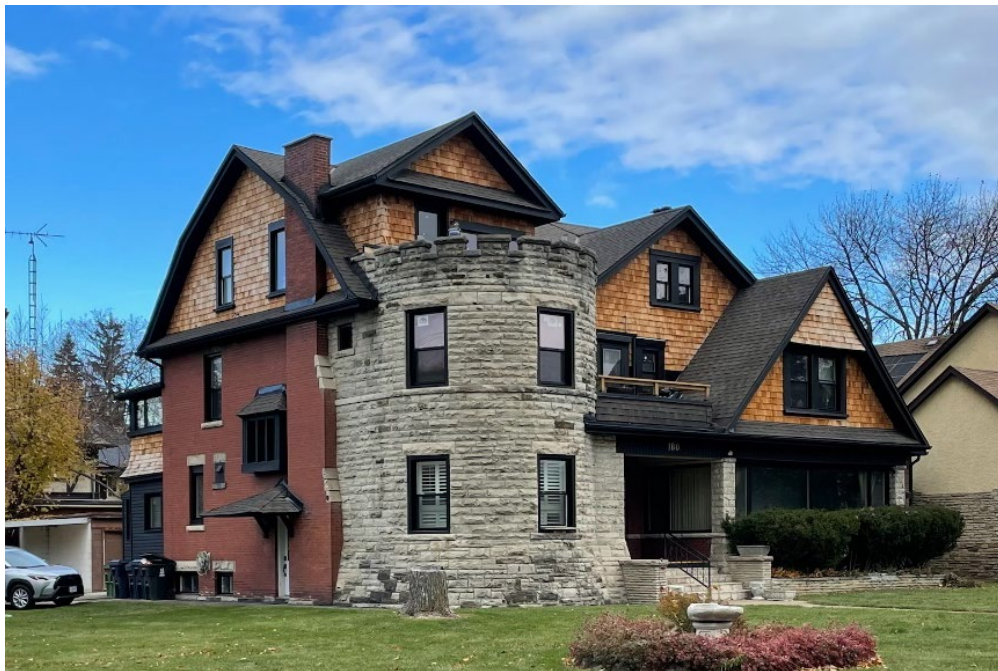
View of 180 Queen's Drive, 2025 (City of Toronto Heritage Planning)
