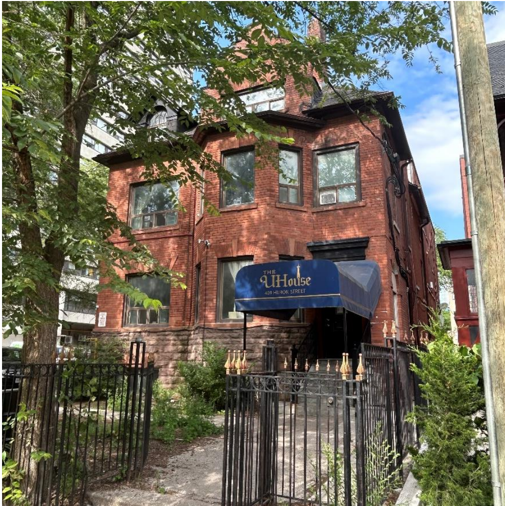
Primary (west) Elevation and partial South Elevation
