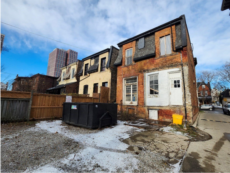
Figure 27. Rear (South) Elevations at 29, 31, and 33 Sussex Avenue showing the parapet walls on the east elevations instead of mansard roofs and the buff brick cladding at 33 and 31 Sussex and, at 29 Sussex, the red wash applied to the rear and side walls (Heritage Planning, 2024)
