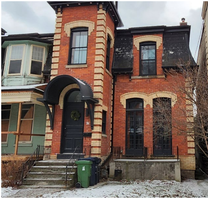
Figure 13. 31 Sussex Avenue showing the mansard roof, the paired French doors, the decorative yellow brick trim with the yellow brick chaine at the corners (Heritage Planning, 2024)
