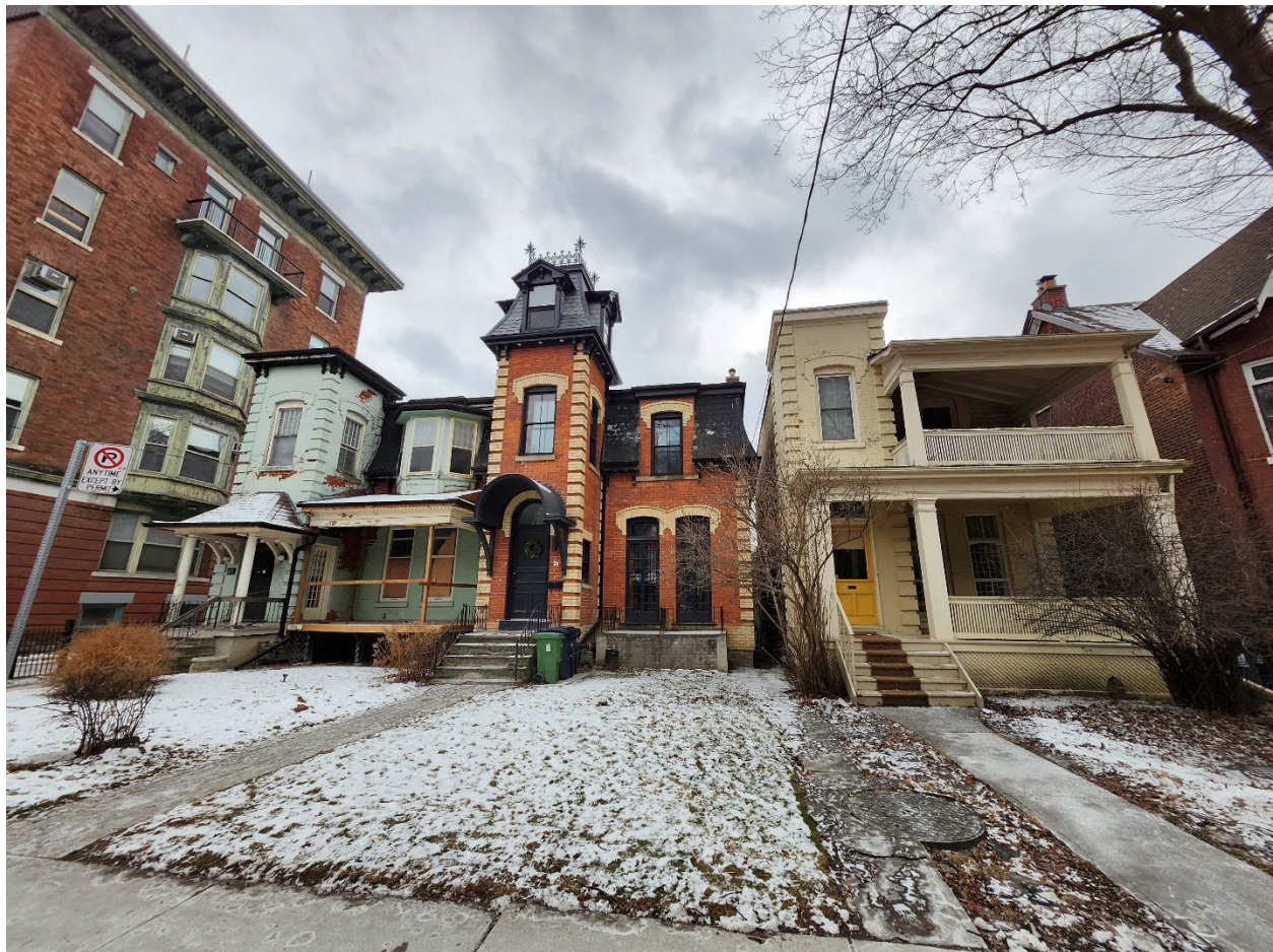
Detail of the principal (north) elevations of 29, 31 and 33 Sussex Avenue (Heritage Planning, 2024)
