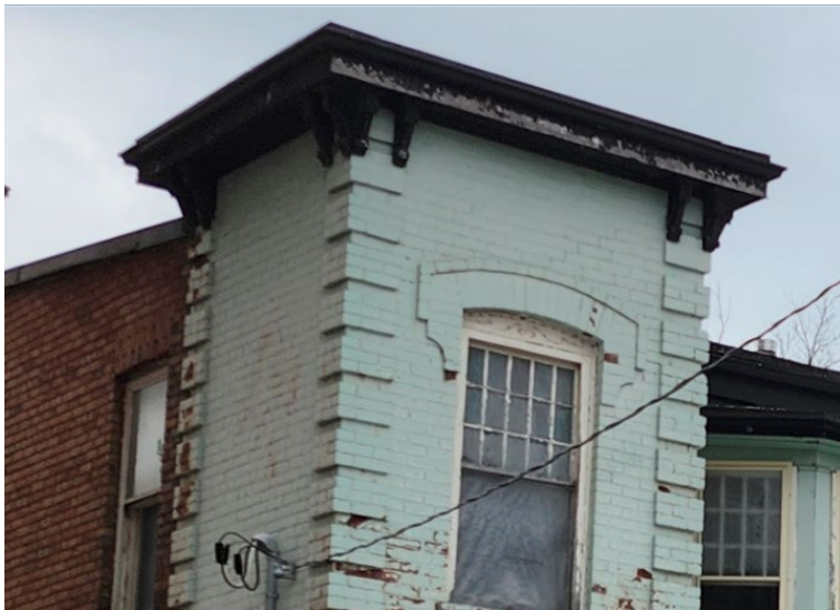
Figure 15. 29 Sussex Avenue showing the details on the tower including the chaine at the corners, the pierced wood lintel over the windows and the paired brackets at the eaves (Heritage Planning, 2024)
