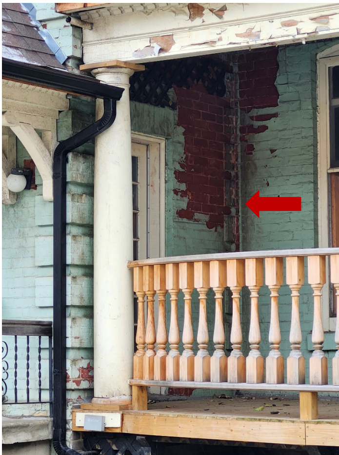
Figure 18. 29 Sussex Avenue showing the chaine extending to the tower return (Heritage Planning, 2024)
