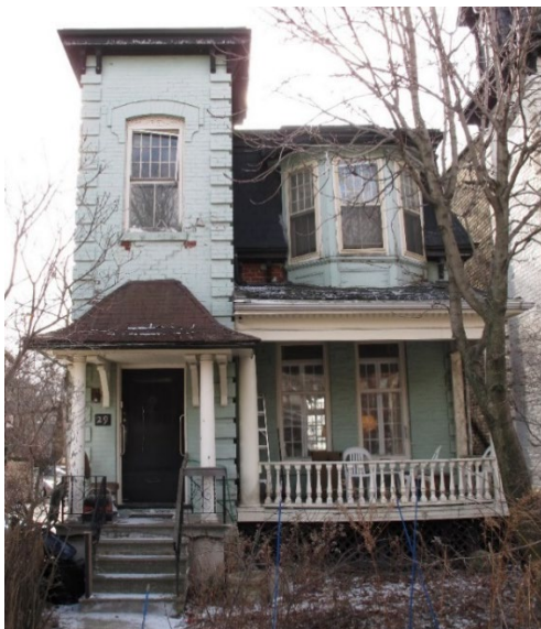
Figure 6. 29 Sussex Avenue (ERA Architects, Inc., 2013)
