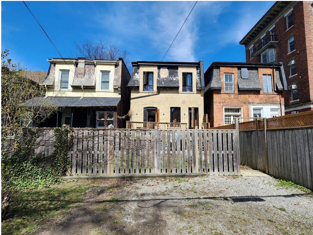
Figure 26. Rear (South) Elevations at 33, 31 and 29 Sussex Avenue showing the mansard roofs on the west and south elevations and the parapet wall on the east (Heritage Planning, 2024)
