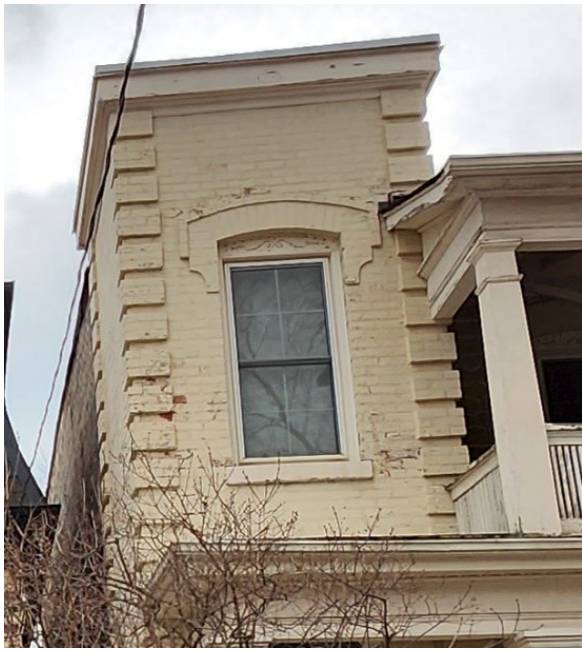
Figure 17. 33 Sussex Avenue showing the chaine at the corners the decorative brick detailing of the segmental arched window opening and the decorative piercing pattern in the wood lintel over the window (Heritage Planning, 2024)
