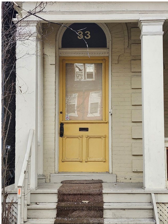
Figure 24. 33 Sussex Avenue showing the door with its panelling and hardware, decoratively carved lintel, and the fanlight (Heritage Planning, 2024)
