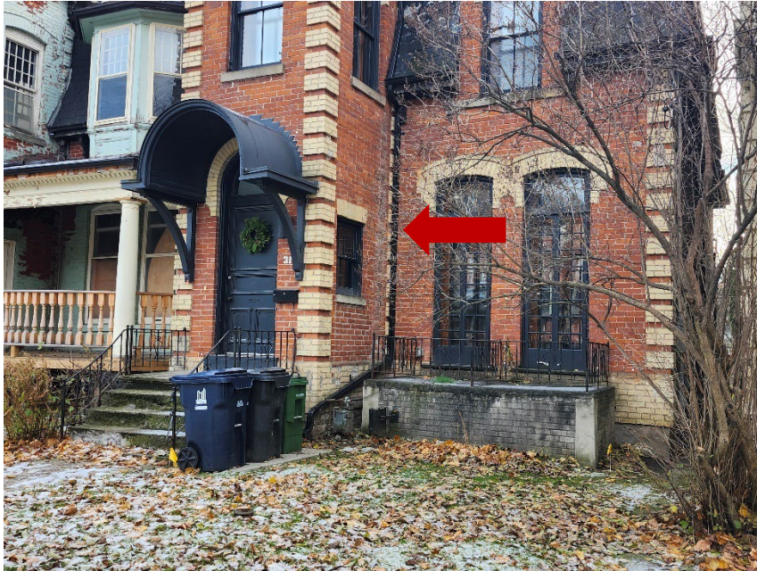
Figure 19. 31 Sussex Avenue showing the chaine extending to the tower return (Heritage Planning, 2024)
