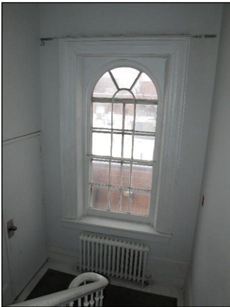
Figures 26 and 27: Left: Interior photo of the Italianate influenced round-headed windows in the c. 1855 section's north façade. Right: On the south elevation, in the c. 1855 two-storey projecting tower, are two Italianate influenced round-headed windows.
