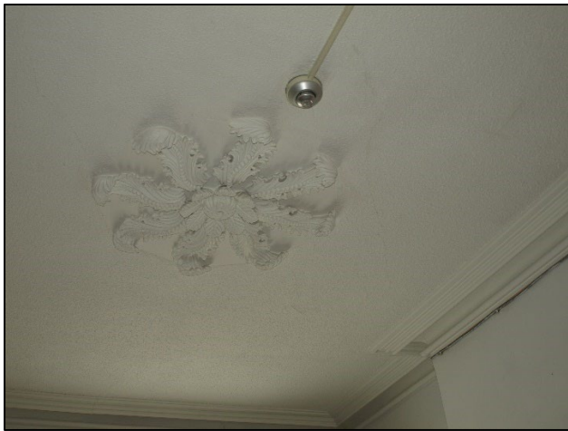
Figure 37: Detail of the plaster medallion and cornice moulding in the c. 1855 section's formal front entry hall. (Heritage Planning, 2025).
