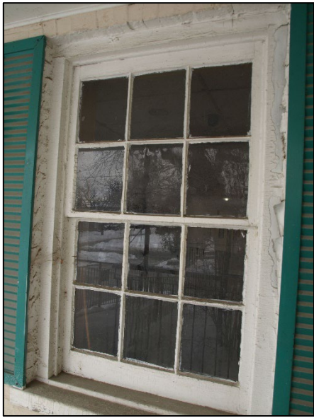
Figures 24 and 25: Left: One of the c. 1843, Georgian influenced section's six-over-six wood windows. Right: one of the c. 1855 Italianate influenced section's round-headed windows on the building's north façade. (Heritage Planning, 2025)
