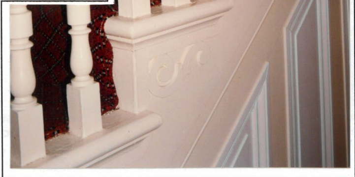
Figure 32: Details showing the c. 1855 formal J-Plan, or double-winder, stairway. (Fayle Associates, 1994)
