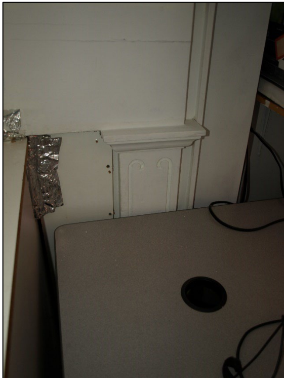
Figures 38 and 39: Hidden fireplaces on the first (left) and second (right) floors. All that is visible is part of the flat pilaster (left) and the corner of the mantel (right) (Heritage Planning, 2025).
