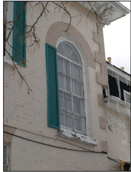
Figures 24 and 25: Left: One of the c. 1843, Georgian influenced section's six-over-six wood windows. Right: one of the c. 1855 Italianate influenced section's round-headed windows on the building's north façade. (Heritage Planning, 2025)
