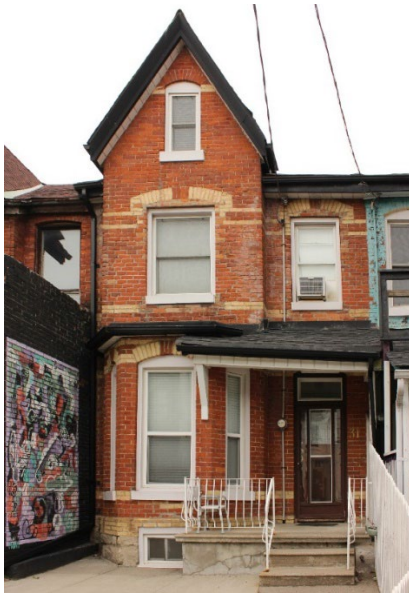
Figure 16. Main (west) façade of 31 Kensington Avenue showing its three-sided ground level bay window and dichromatic brickwork designs (Heritage Planning, 2025).
