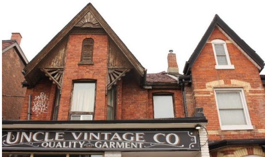
Figure 17. Comparison of the projecting bays and gables at 33 (left) and 31 Kensington Avenue (right) showing their different designs (Heritage Planning, 2025).
