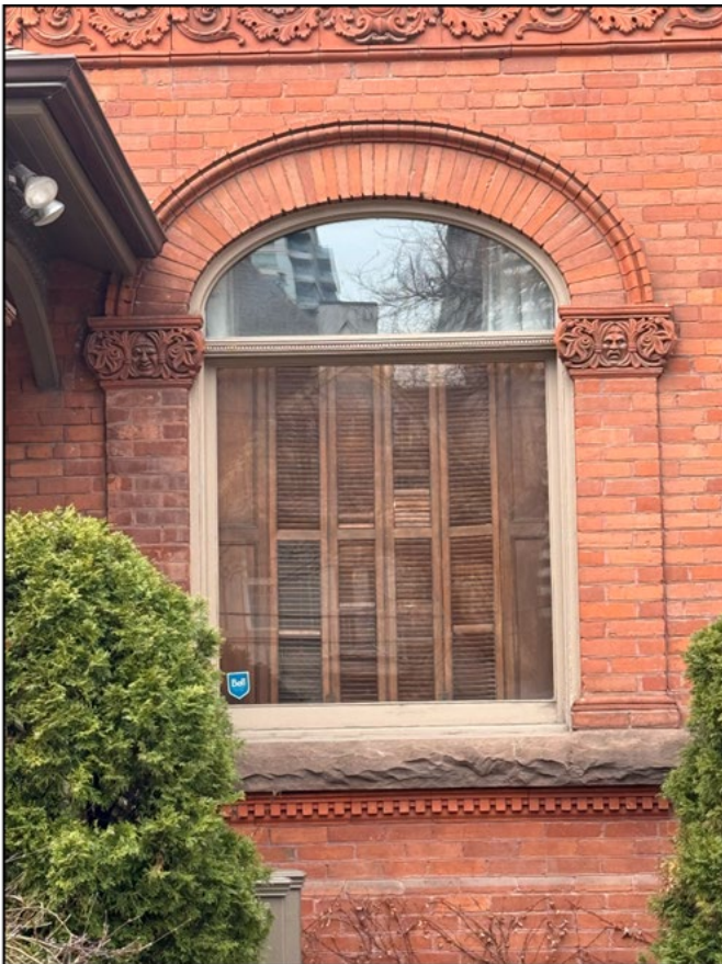
Figure 14. First storey window detail at 506 Jarvis Street showing brick pilasters with terra cotta capitals and beneath a terracotta string course (Alex Corey Heritage Consulting, 2025).
