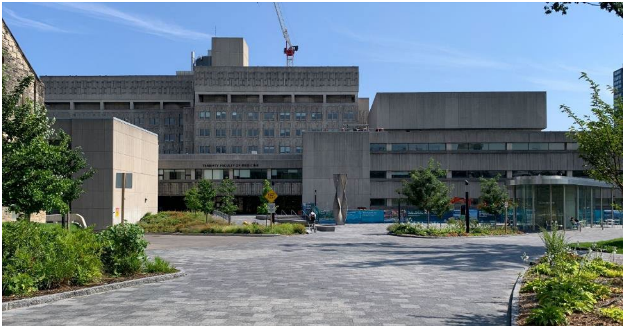
Medical Sciences Building, primary (north) elevation (Heritage Planning, 2025).
