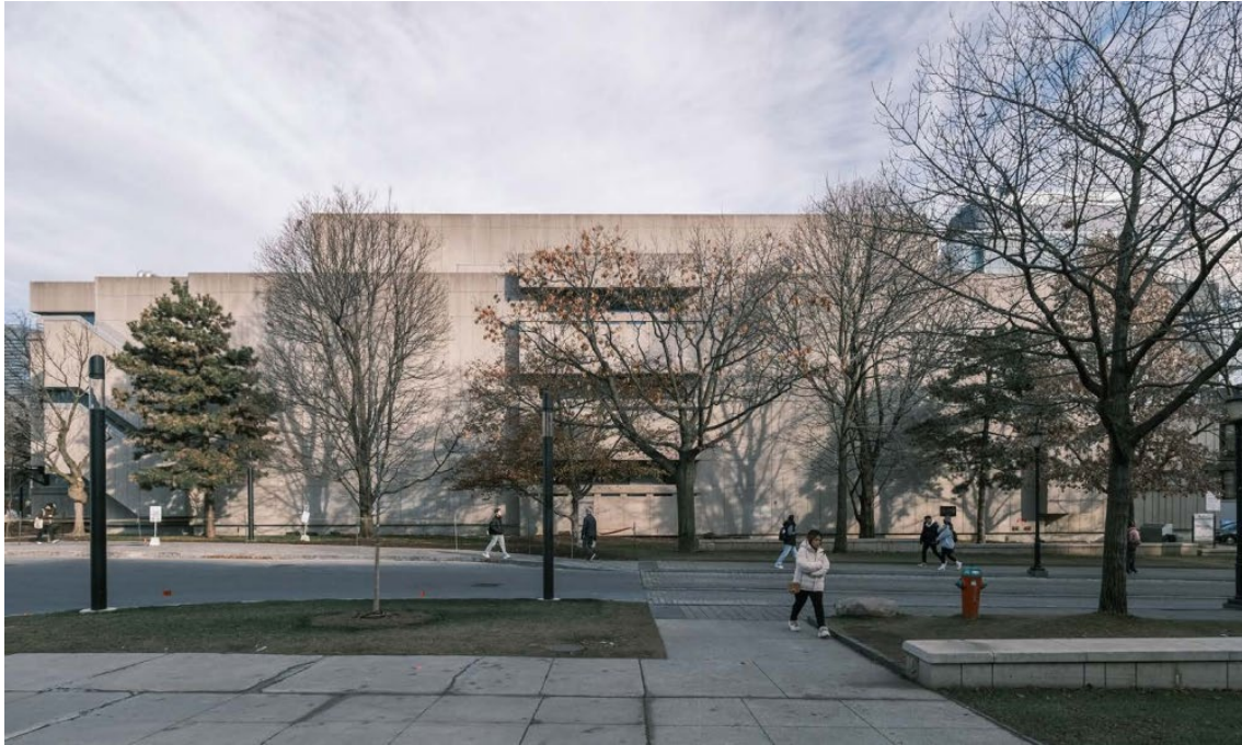
Figure 13: West elevation of west wing, view from across King's College Road (ERA, November 2023).
