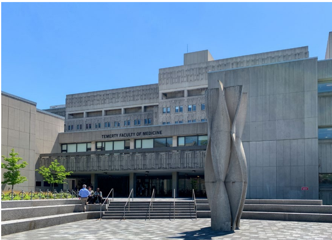
Figure 8: Detail of the main entrance on primary (north) elevation, showing the tiered massings framed by the Macleod Auditorium and stairwell (Heritage Planning, 2025).
