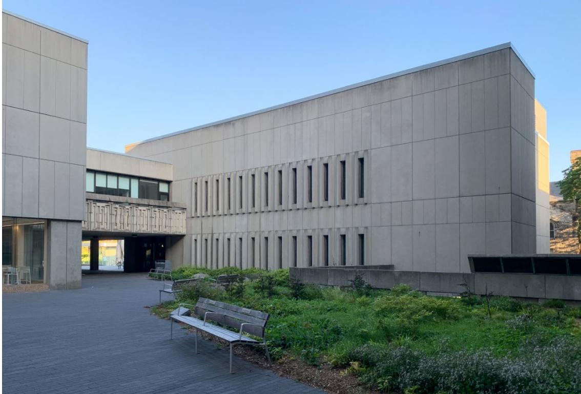
Figure 11: South elevation of Macleod Auditorium, showing the vertically-oriented windows with projecting window fins (Heritage Planning, 2025).
