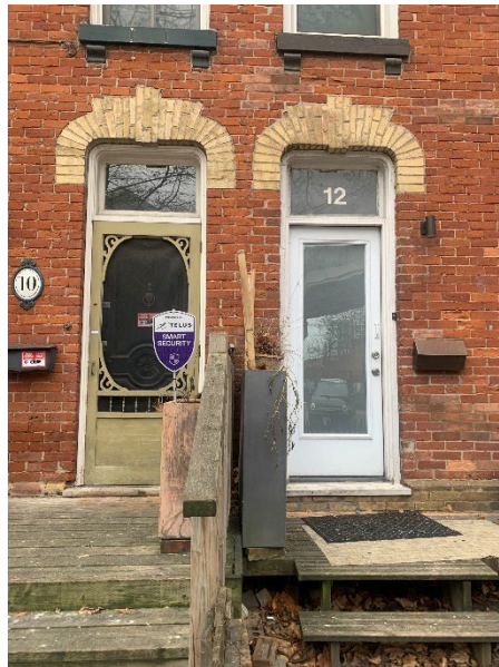
Images 11 and 12: Detail of the principal elevations at 6-8 and 10-12 Sumach Street, showing the decorative contrasting brickwork and original door openings with transoms. The stained glass transom at 8 Sumach Street is likely original to the 1886 house. (Heritage Planning, 2025)
