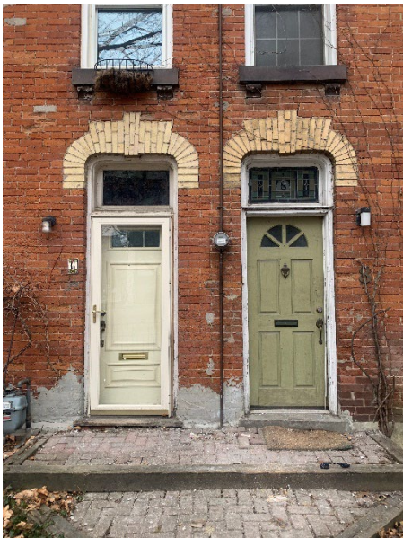
Images 11 and 12: Detail of the principal elevations at 6-8 and 10-12 Sumach Street, showing the decorative contrasting brickwork and original door openings with transoms. The stained glass transom at 8 Sumach Street is likely original to the 1886 house. (Heritage Planning, 2025)
